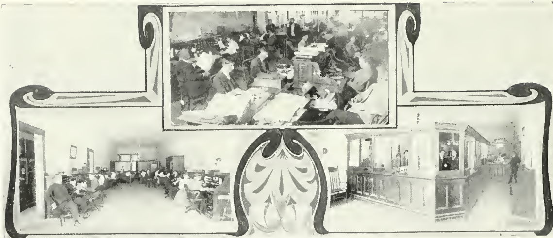
Interior Views, Offices of Company, 335-337 South Hill Street, Los Angeles, Cal.
