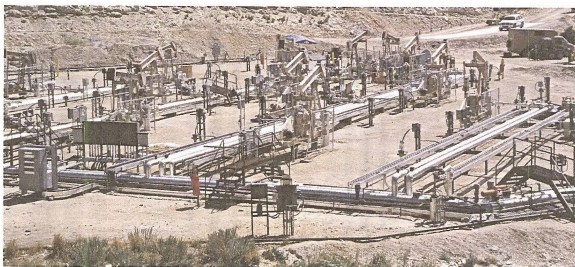
FIGURE A-8 Shell's Field Research in Rio Blanco County, Colorado (Courtesy: Shell Exploration & Production; reprinted with permission.)
