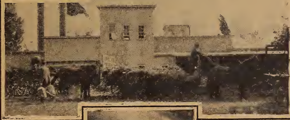
A pan evaporator over a fire arch, housed in a building typical of the old-fashioned sorghum-sirup plant
