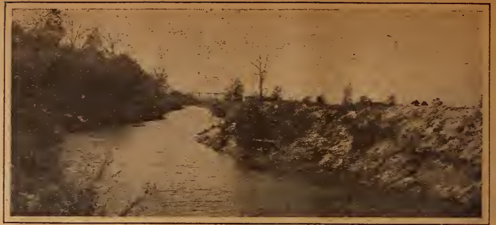
A 40-mile ditch in Daviess County, Indiana, that has changed a lot of water-soaked land into fertile farms
