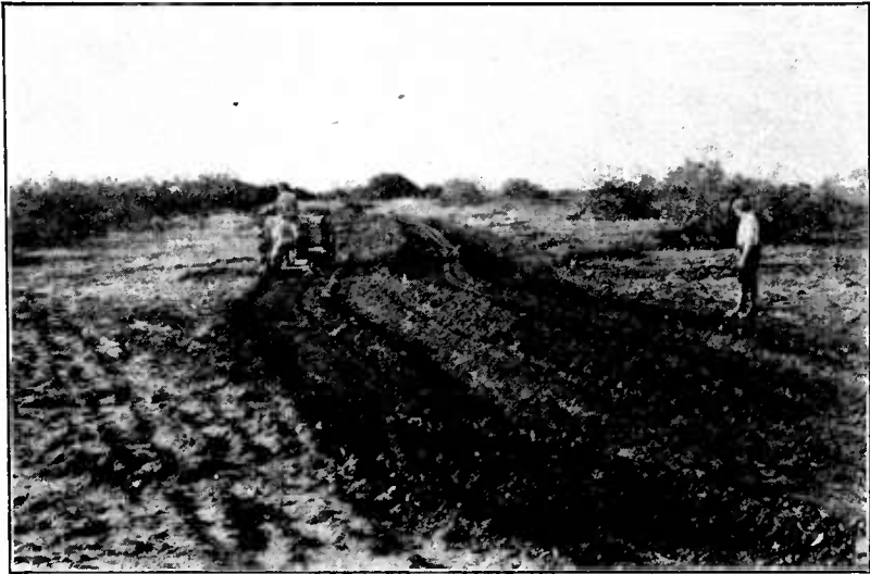
FIGURE 19.—Building a terrace with a single-blade steel terracing machine. The machine is cutting dirt to be moved toward the center of the terrace on the next round
