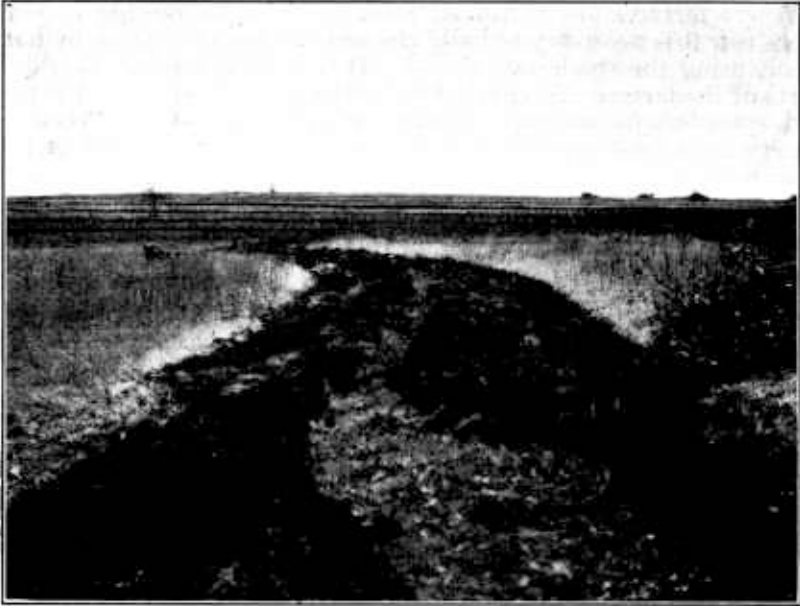
FIGURE 18.—One method of starting the construction of a terrace with the single-blade terracing machine shown in Figure 15. One round with the machine has been made, the furrows being about 8 feet apart
