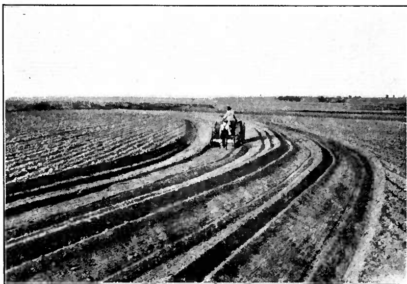
FIGURE 20.—Building a terrace with a single-blade terracing machine. The machine is moving dirt toward the center of the terrace
