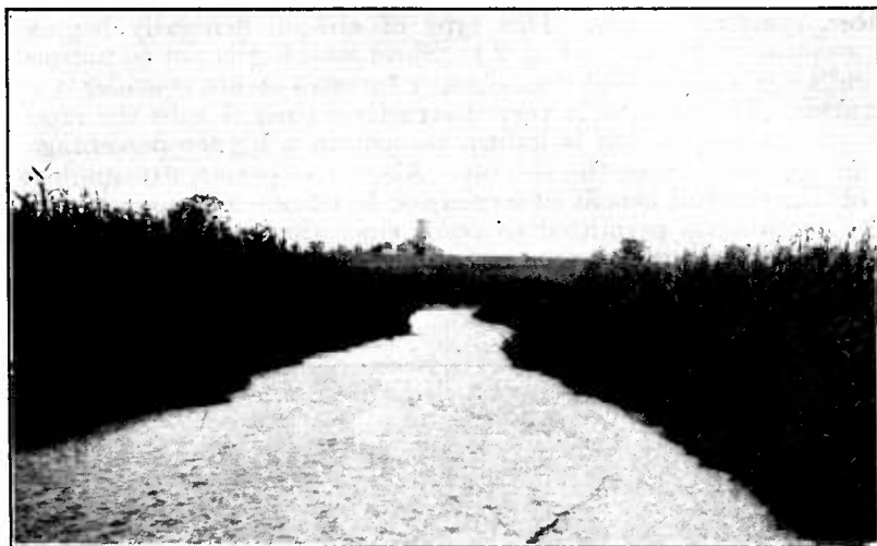
FIGURE 3.—Drainage ditch partly filled with sand washed from eroding hills
