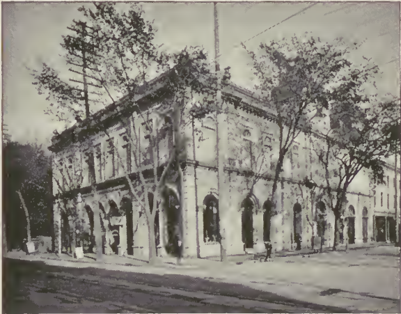
THE ART ASSOCIATION BUILDING, MONTREAL.
