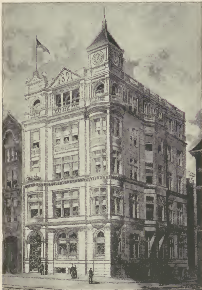
BUILDING AND HEAD OFFICE OF THE SUN LIFE ASSURANCE COMPANY OF CANADA.
