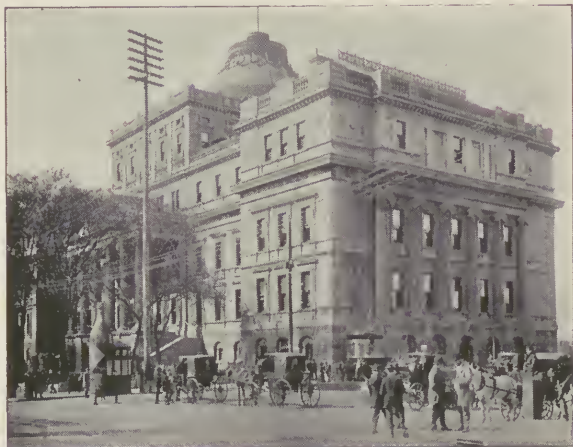
COURT HOUSE, MONTREAL.
