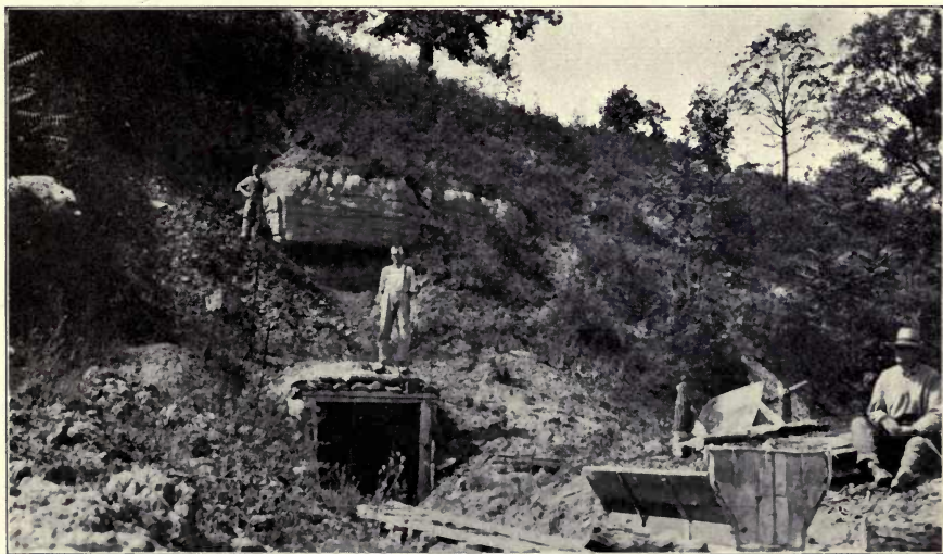
B—The Carl Crabtree mine in which Tionesta clay is mined for the general market. Putnam Hill limestone exposed about 15 feet above the mine. Blunt Run, Muskingum County (Locality 27)
