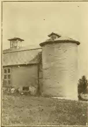
Round Silo Built of Shiplap.
