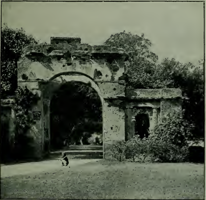
THE GATEWAY OF THE RESIDENCY, LUCKNOW, SHOWING MARKS OF SHOT AND SHELL ON THE BRICKWORK.
