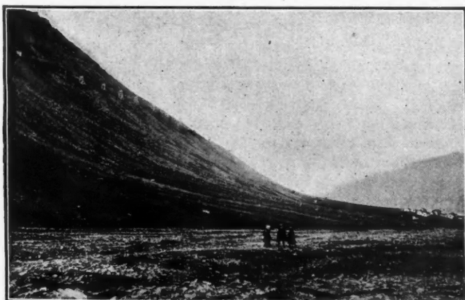
SIDE VIEW OF THE AERIAL TRAMWAY, SHOWING BARREN CHARACTER OF LAND
