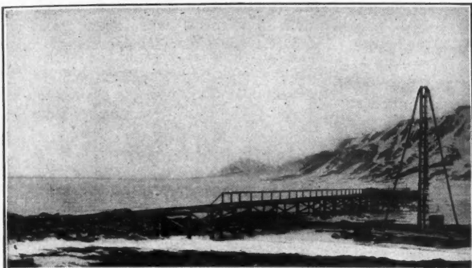
THE LANDING STATION WHERE CONSTRUCTION MATERIALS WERE FIRST LANDED
