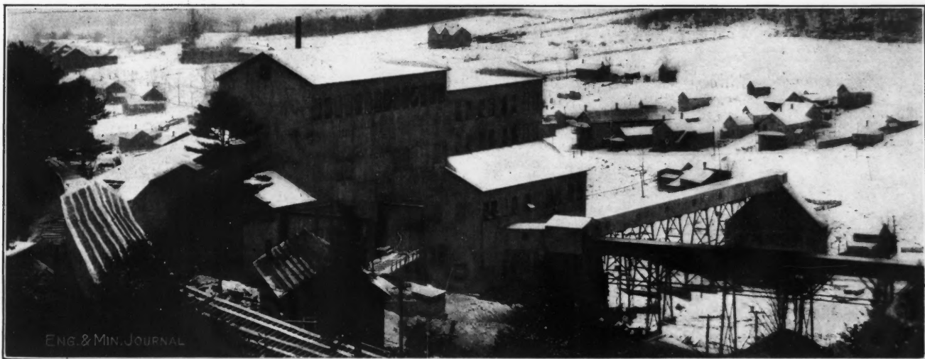
MILL LOOKING SOUTHEAST FROM BARTON HILL WITH COVERED TRACK FROM MINE. NOTE HOUSED CONVEYOR TO SHIPPING BINS ON RIGHT
