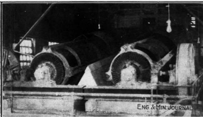
TROMMELS OF SEPARATING DEPARTMENT. DRIER STACK IN BACKGROUND
