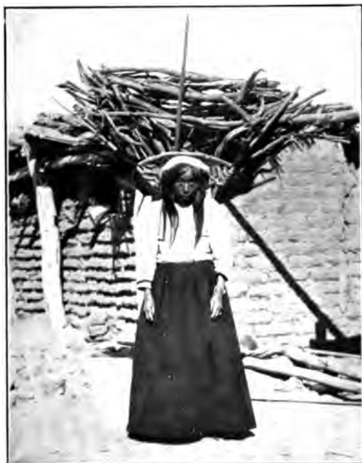
c THE LOAD IN POSITION
