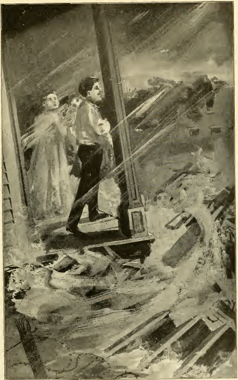
DESTRUCTION OF HOMES BY THE GALVESTON STORM
