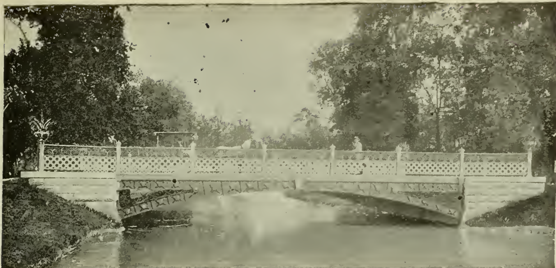
FIG. 1.—BRIDGE OVER CANAL, BELLE ISLE PARK, DETROIT.
