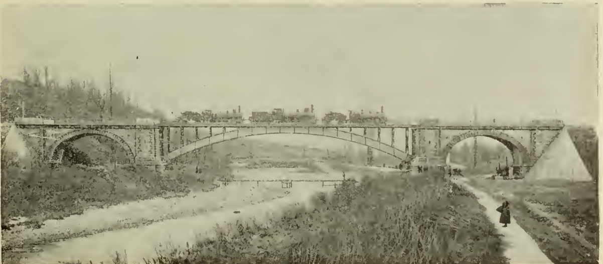
FIG. 3.—RAILROAD BRIDGE NEAR LOERRACH, BADEN.
