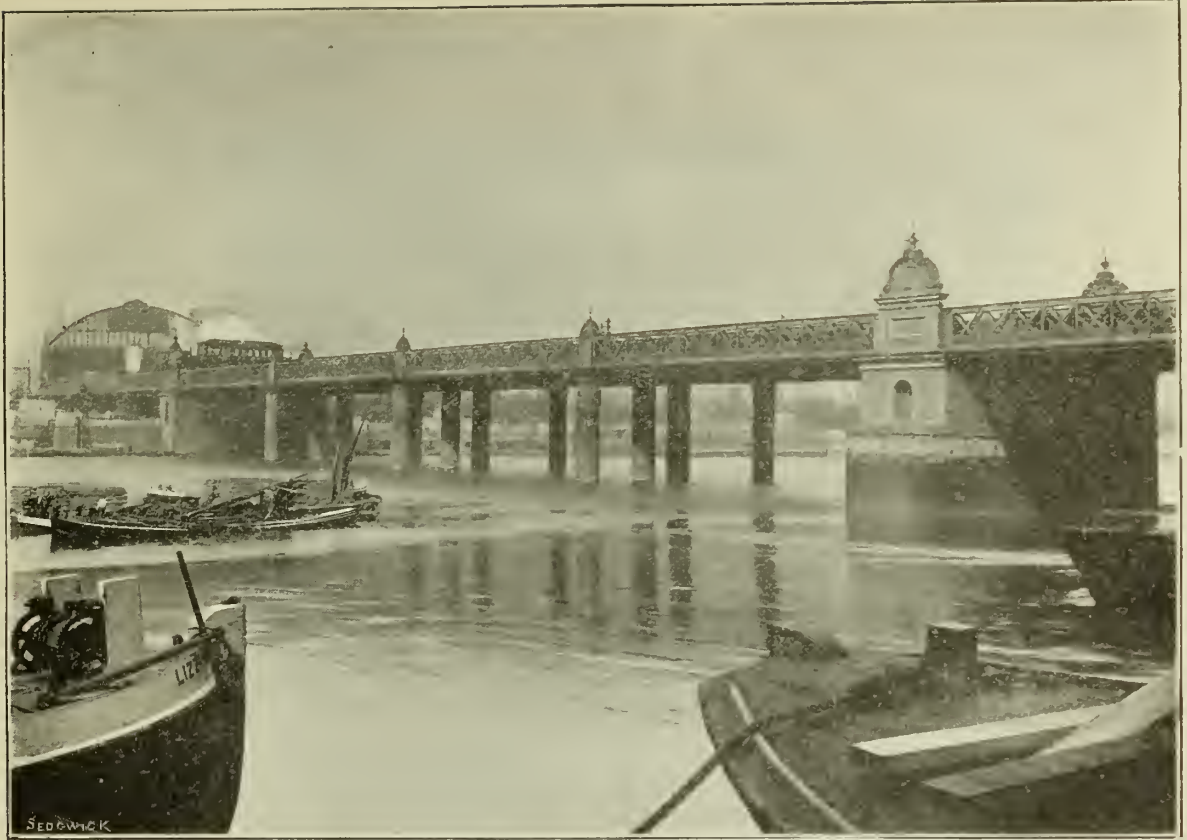
FIG. 1.—CHARING CROSS RAILWAY BRIDGE, LONDON.
