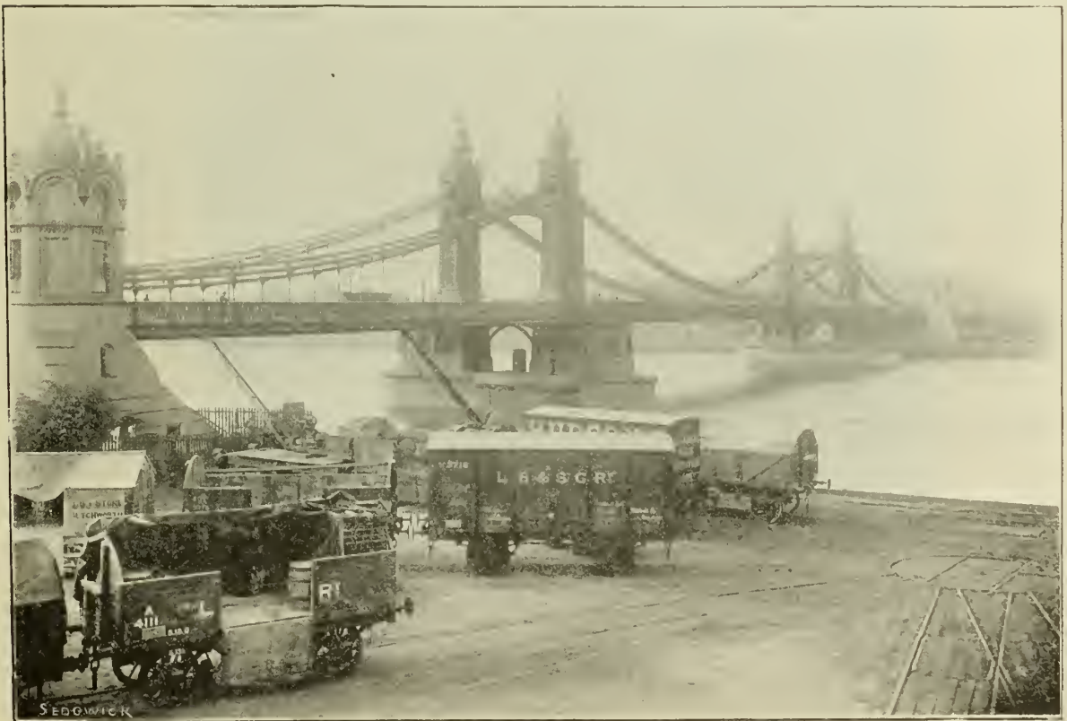
FIG. 2.—THE VICTORIA BRIDGE, LONDON.
