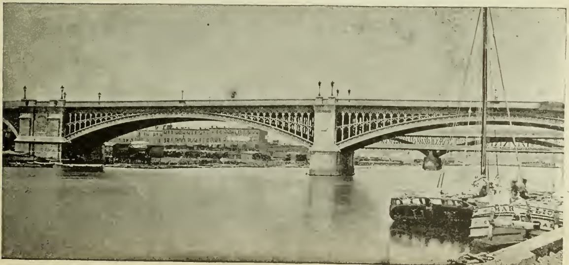
FIG. 3.—CHESTNUT STREET BRIDGE OVER SCHUYLKILL RIVER, PHILADELPHIA.
