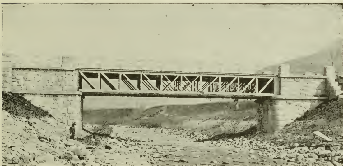
FIG. 2.—HIGHWAY BRIDGE OVER WEHRA RIVER, WEHR, BADEN.
