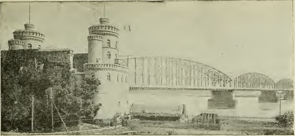
FIG. 1.—RAILROAD BRIDGE OVER THE RHINE AT MAYENCE, GERMANY.
