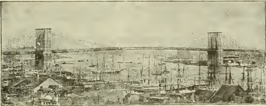
FIG. 3.—NEW YORK AND BROOKLYN SUSPENSION BRIDGE.
