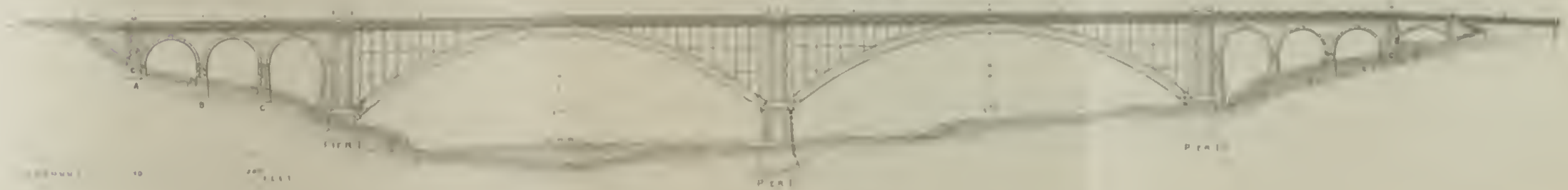
THE HARLEM RIVER BRIDGE AS BUILT (NOW CALLED WASHINGTON BRIDGE)
