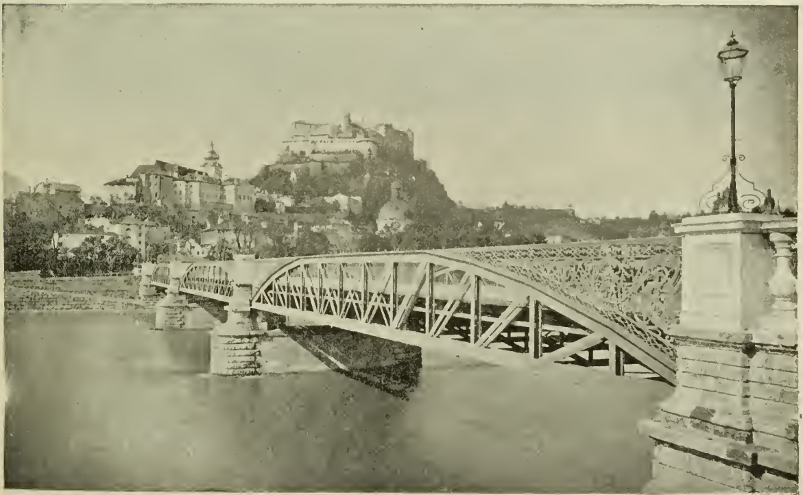
FIG. 2.—METAL BRIDGE OVER INN RIVER IN SALZBURG, TYROL.
