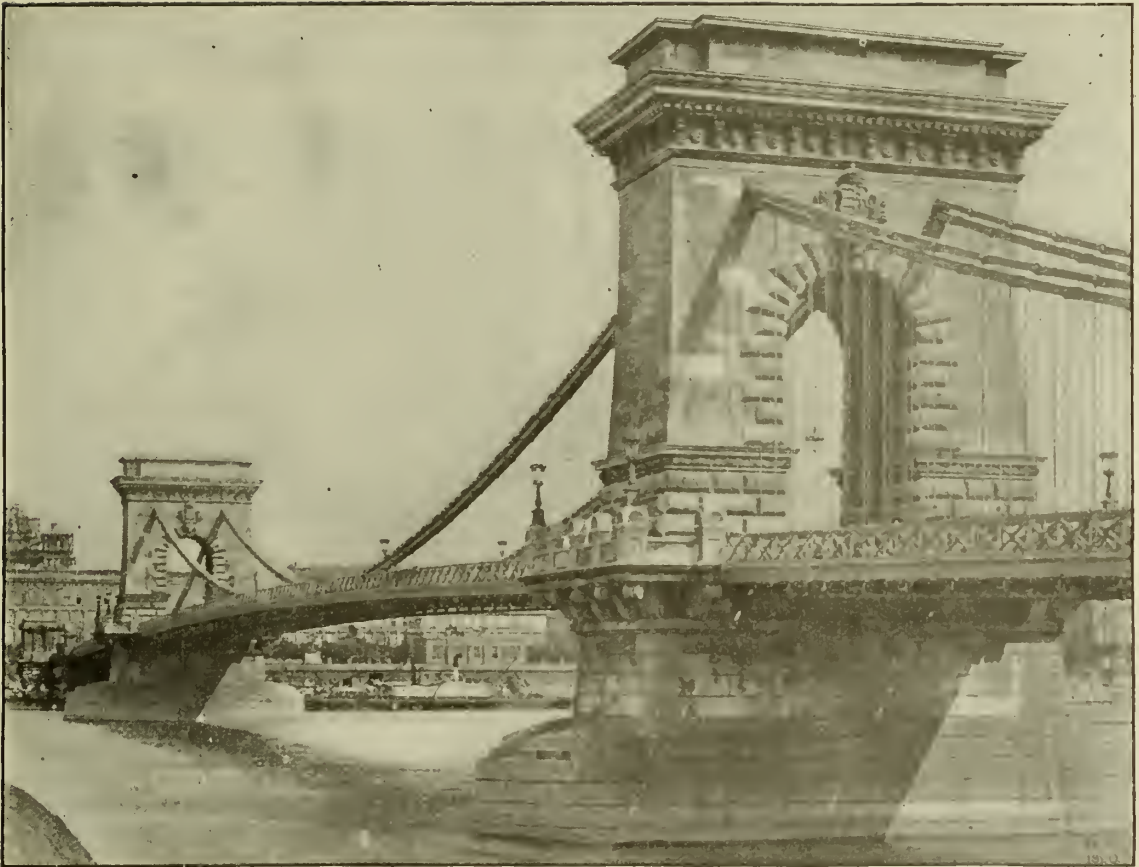
BUDA-PESTH SUSPENSION BRIDGE.
