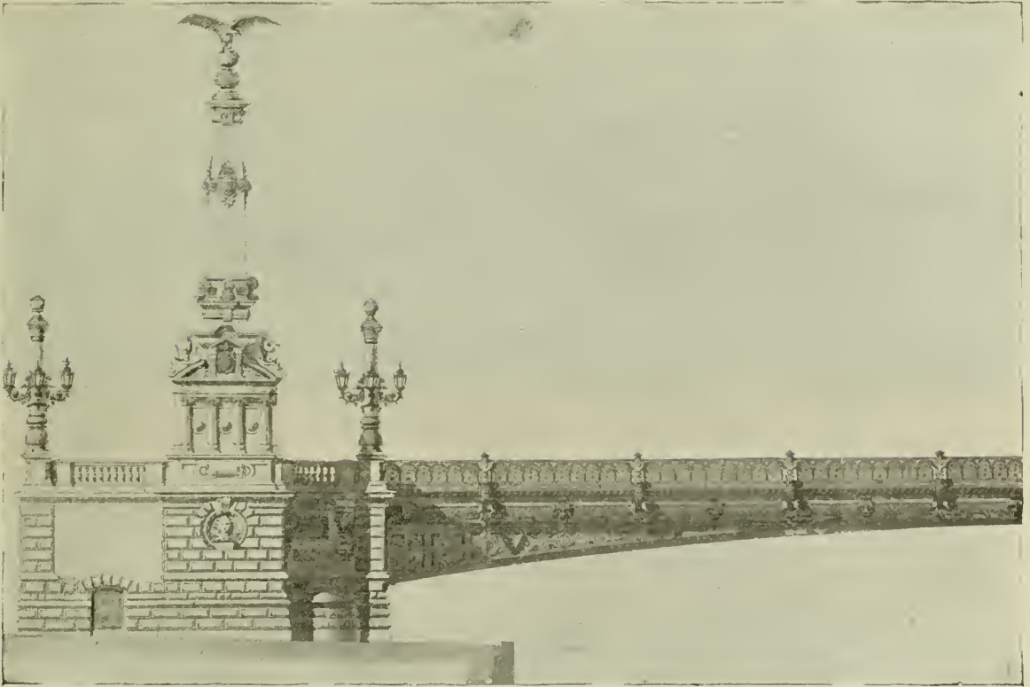
FIG. 1.—STEPHANIE BRIDGE OVER DANUBE CANAL IN VIENNA.
