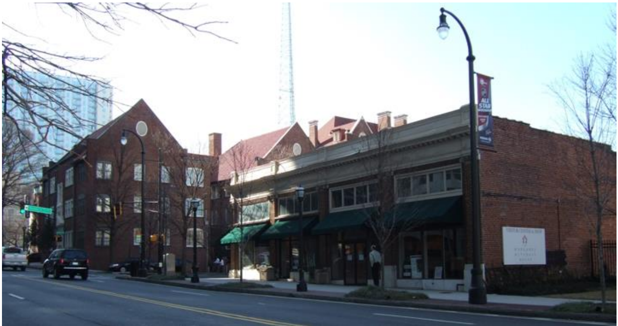
Commercial Row looking south along Peachtree Street, 2008
