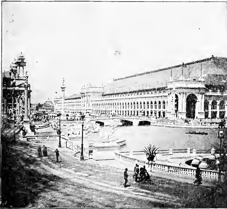
WEST SIDE OF MANUFACTURES AND LIBERAL ARTS BUILDING.
