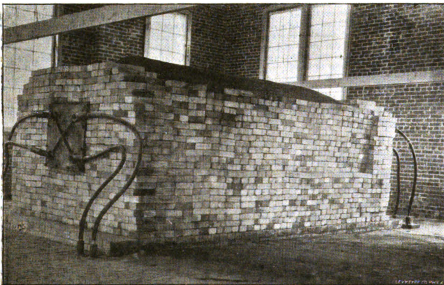
FIG. 1.—Carborundum furnace ready for operation.
