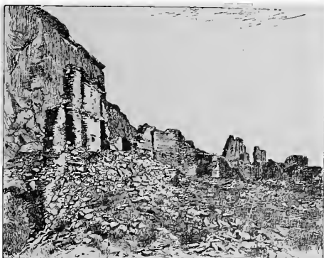
RUINED HOUSE IN CHACO CANYON.
