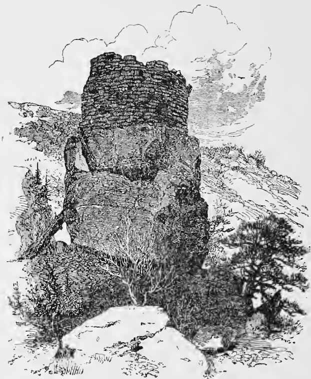
FIG. 2. BLACK TOWER ON THE MANCOS
