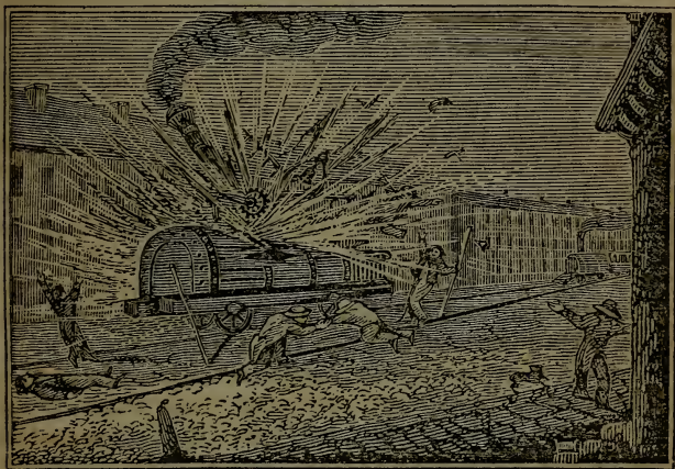
Explosion of a locomotive on the Harlaem railroad.
