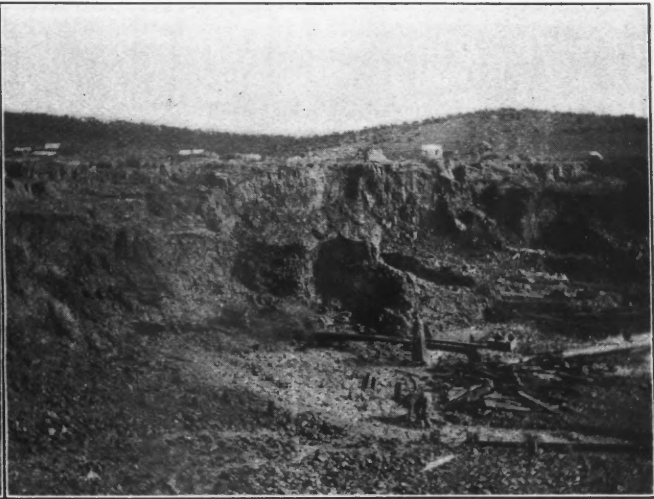
FIG. 2. SLUICING WITH ARTIFICIAL HEAD.
