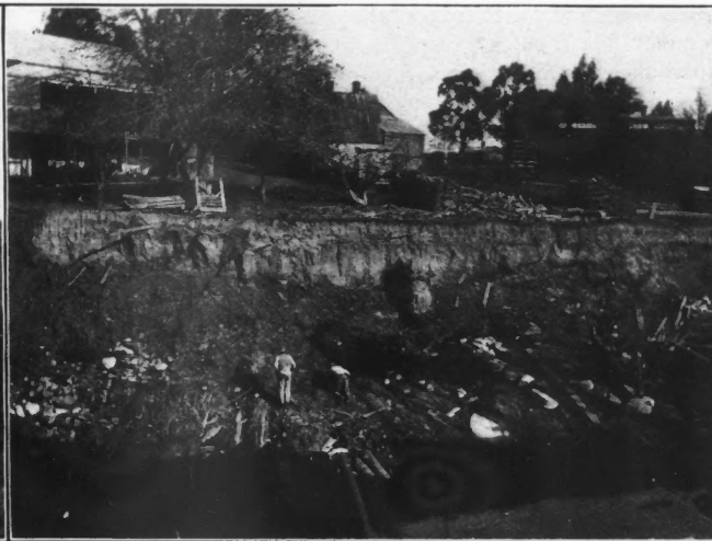
FIG. 7. CLEANING UP BED-ROCK.
