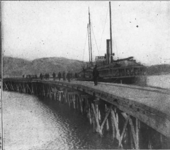
UNLOADING RAILS FOR ALASKA CENTRAL RAILWAY AT SEWARD.
