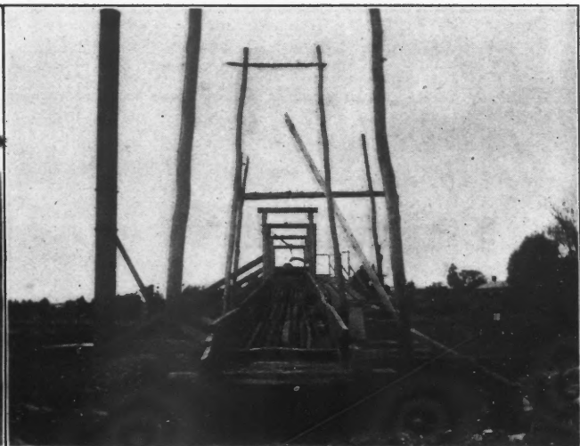
FIG. 6. VIEW UP SLUICE BOX.
