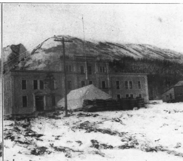
ALASKA CENTRAL OFFICE BUILDINGS DURING CONSTRUCTION.
