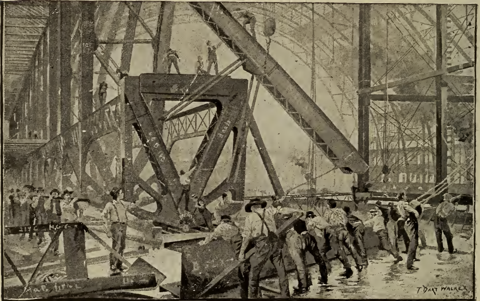
ERECTION OF MANUFACTURES BUILDING.
