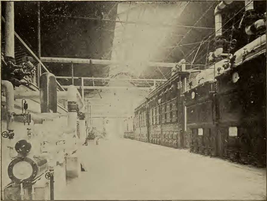
THE BOILERS IN MACHINERY HALL.
