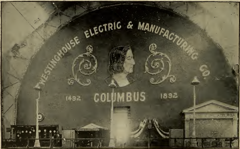
MURAL DECORATION IN EXHIBIT OF WESTINGHOUSE ELECTRIC COMPANY.
