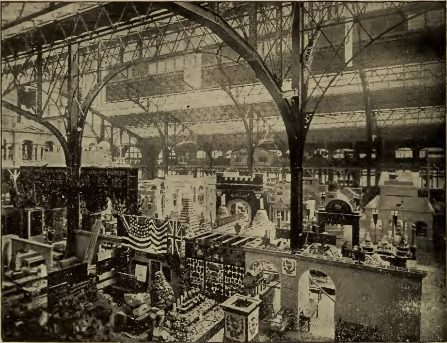
VIEW IN NORTH END OF BUILDING.
