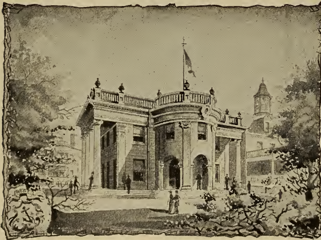
RHODE ISLAND STATE BUILDING.
