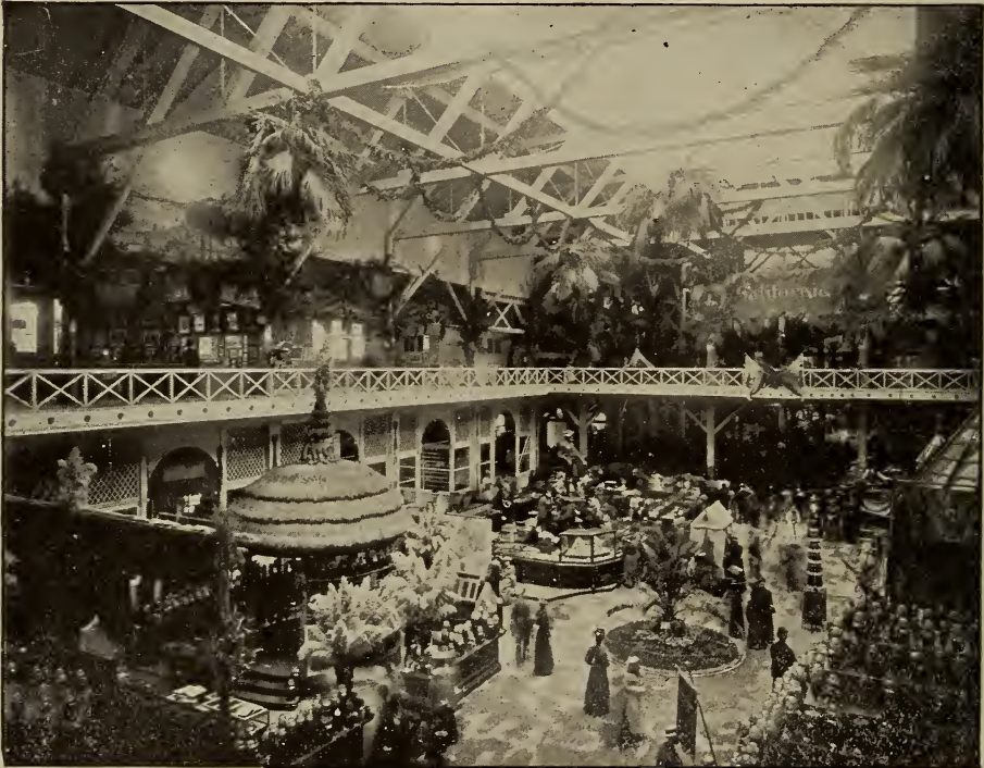
INTERIOR OF CALIFORNIA BUILDING.
