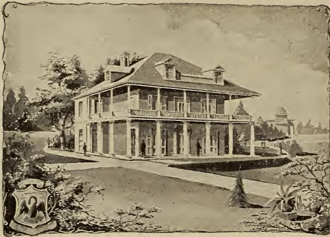
LOUISIANA STATE BUILDING.
