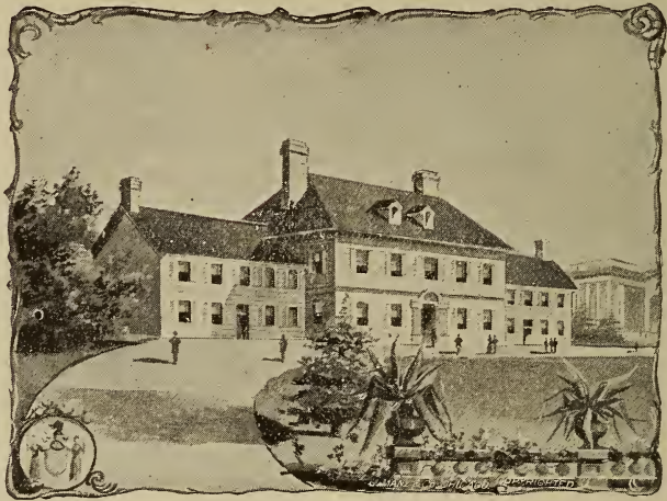
NEW JERSEY STATE BUILDING.
