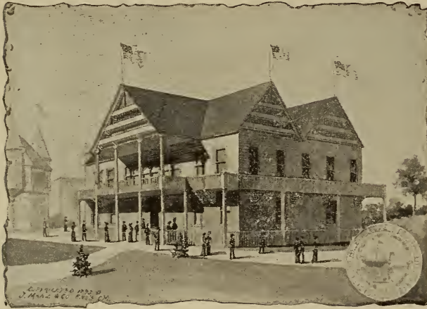
NEW HAMPSHIRE STATE BUILDING.
