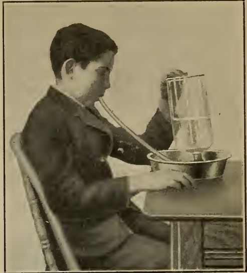
FIG. 96. — Measuring the capacity of the lungs. The bottle was filled with water, which is being forced out by expiring the air from the lungs through the rubber tube slipped up into the mouth of the bottle kept under water in the pan.
