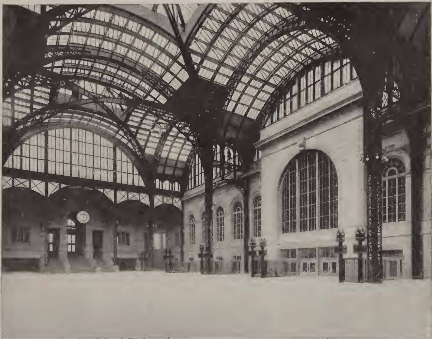
CONCOURSE SHOWING TRAIN GATES AND INDICATORS
