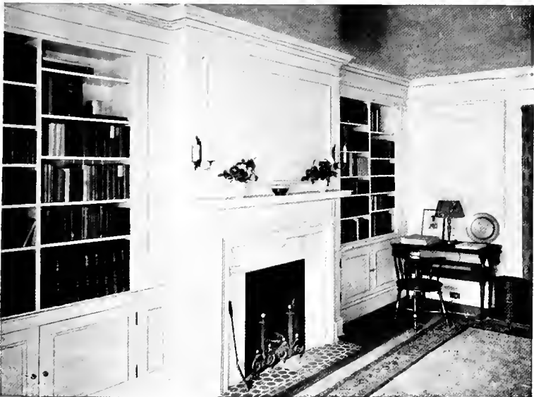
B. WALLS COVERED WITH FILLED CANVAS, AND MOULDING APPLIED TO FORM PANELS
