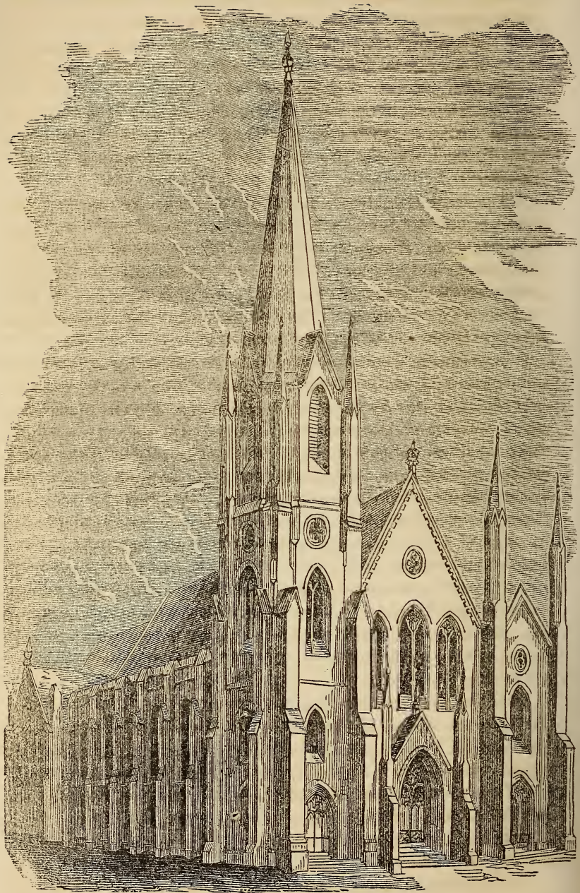
PRESBYTERIAN CHURCH, FIFTH AVENUE AND NINETEENTH STREET, NEW-YORK.
