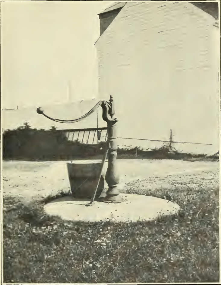
A. WELL AT COUNTY JAIL, WISCASSET. Showing best method of protection from surface drainage.
