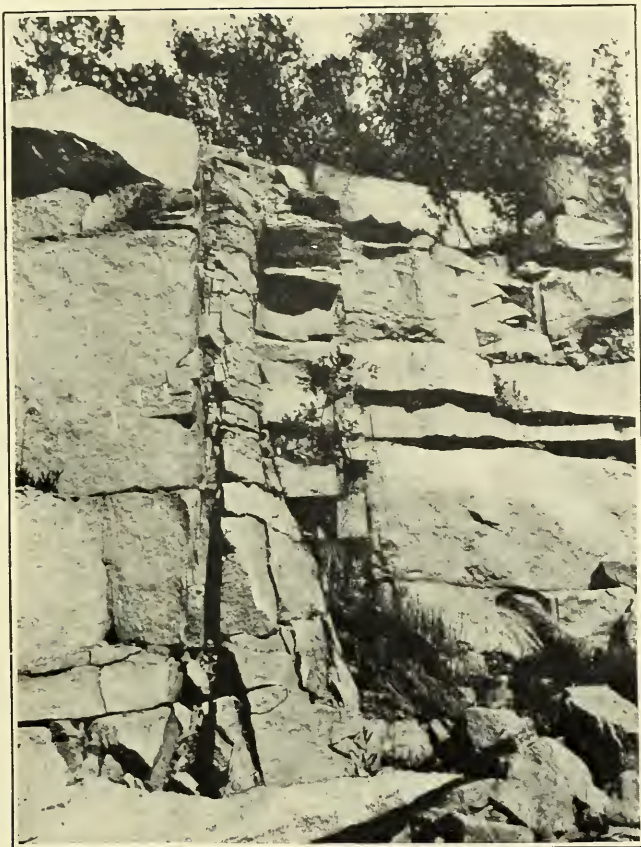
A. ZONE OF NEARLY VERTICAL JOINT CRACKS IN GRANITE QUARRY.
