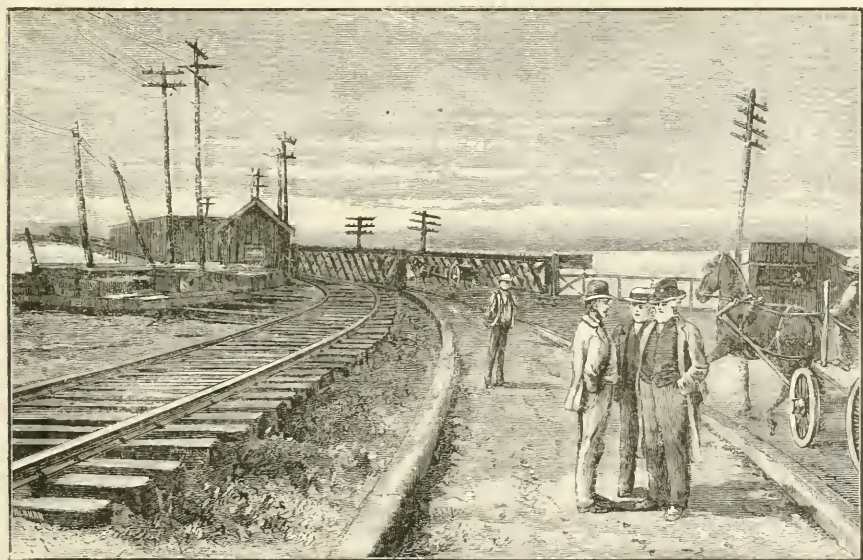
ENTRANCE TO LONG BRIDGE.
