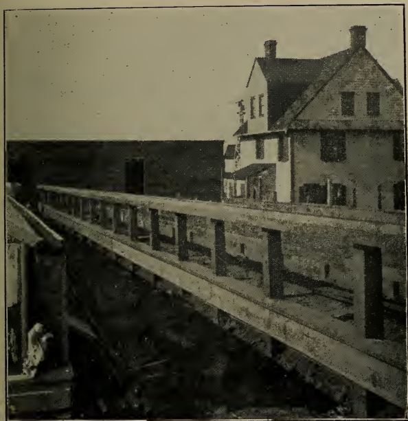
24.—Constructing house twenty-four feet wide; third step, running gutters and notching plate around posts.
