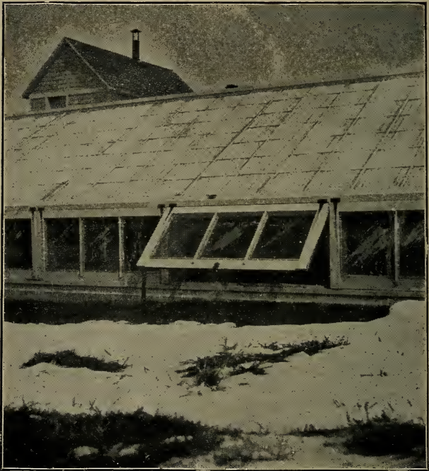
13.—A twelve foot house, showing method of constructing and attaching side ventilators.
