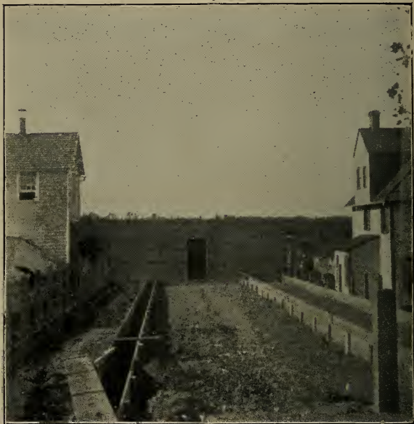
23.—Constructing house twenty-four feet wide; second step, making beds and walks.
