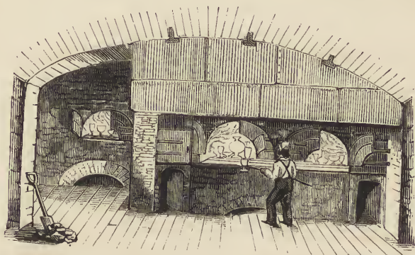
Front view of the annealing arches, showing three sets of pans heating each with a separate fire, with the same cylindrical brick arches and cast-iron doors
