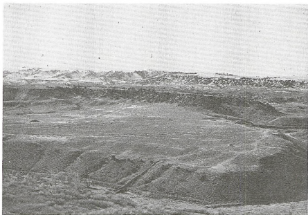
Figure 5.10-A South dam abutment and emergency spillway area.
