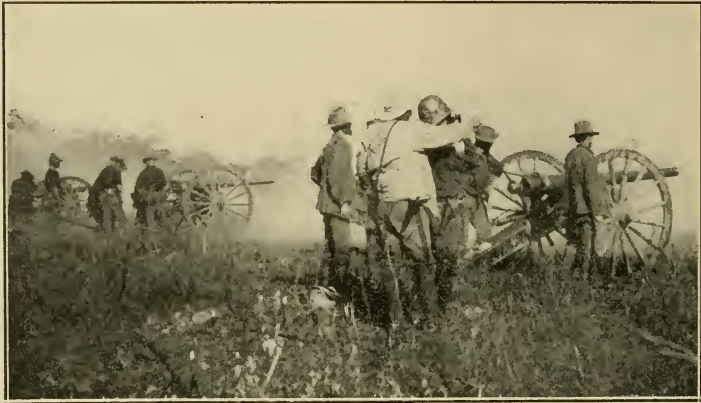
Battery in Action.
