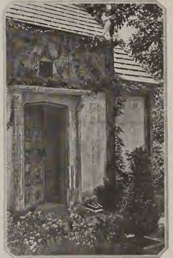
A quaint entrance was made with an old carved wood paneled door and an old stone architrave. To make this Tudor door the architect used old stone fragments and two stone heads. A candle fixture set in the little window above lights the doorway and vestibule
