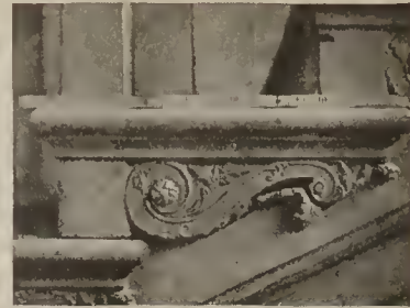
Bracket under treads at State House, Philadelphia
