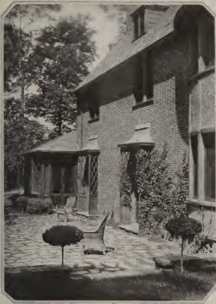
Early English in style, the house has been cleverly adapted to its surroundings. It is of red brick with natural finish oak trim. The south terrace, looking west, shows broken slabs with sod joints. The quaint hood and lattice round the French windows add an old-world touch
