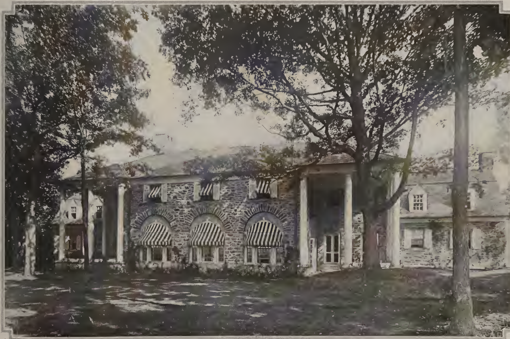
The house was designed and built to accommodate guests fond of outdoor life and for entertaining during the winter hunting season. It is of field stone set in wide white bond, with white wood trim. The roof is shingle
