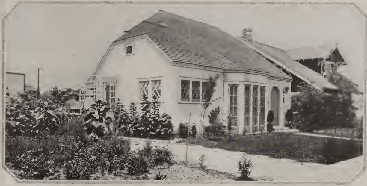
The roof and the window frames as well as the doors are apple green, with yellow flowers planted nearby and hollyhocks underneath the windows
