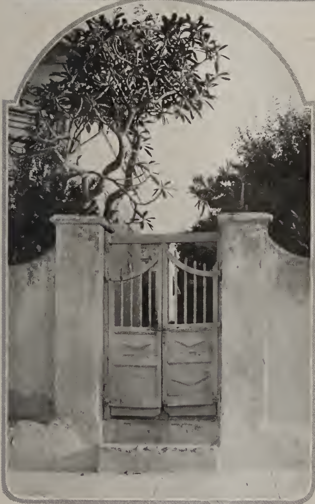
In Bermuda the most prevalent use of whitewash is found. The coral rock walls regularly receive their annual coat, the wash being tinted pink or blue or yellow
