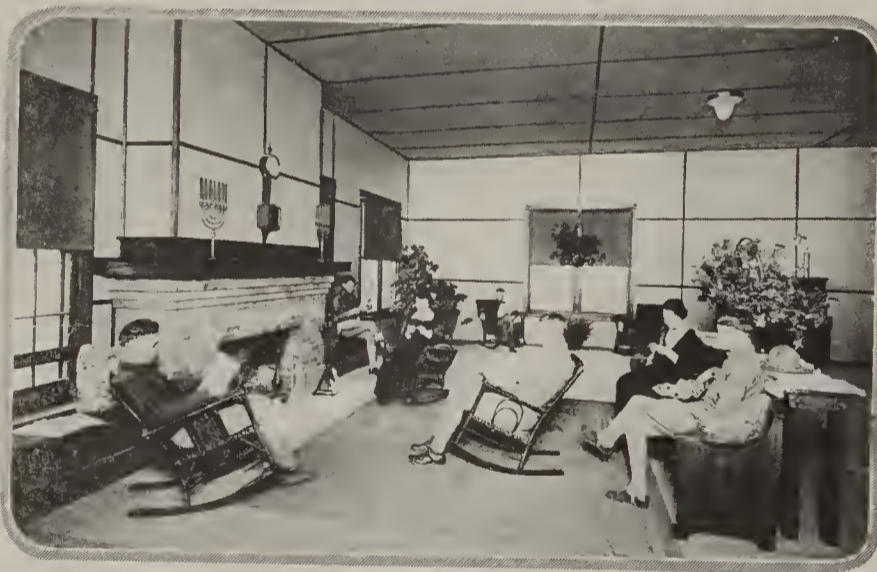
At Camp Travis, Texas, the hostess house living room has walls of wall board and strips
