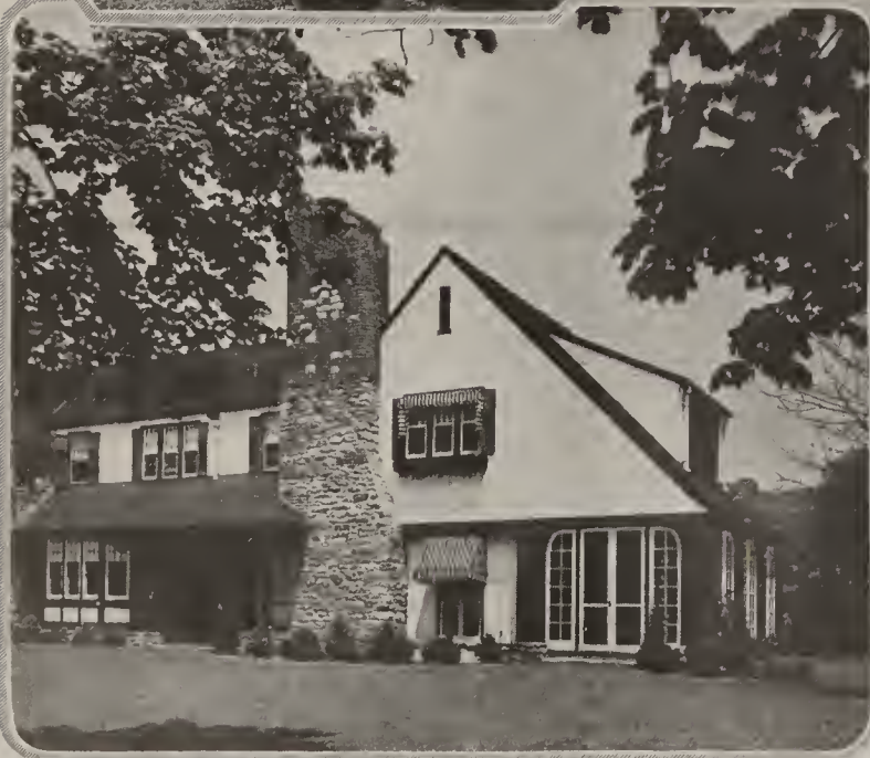
The walls are rubble with a heavy coating of white-wash, a combination that gives interesting light and shade effects
