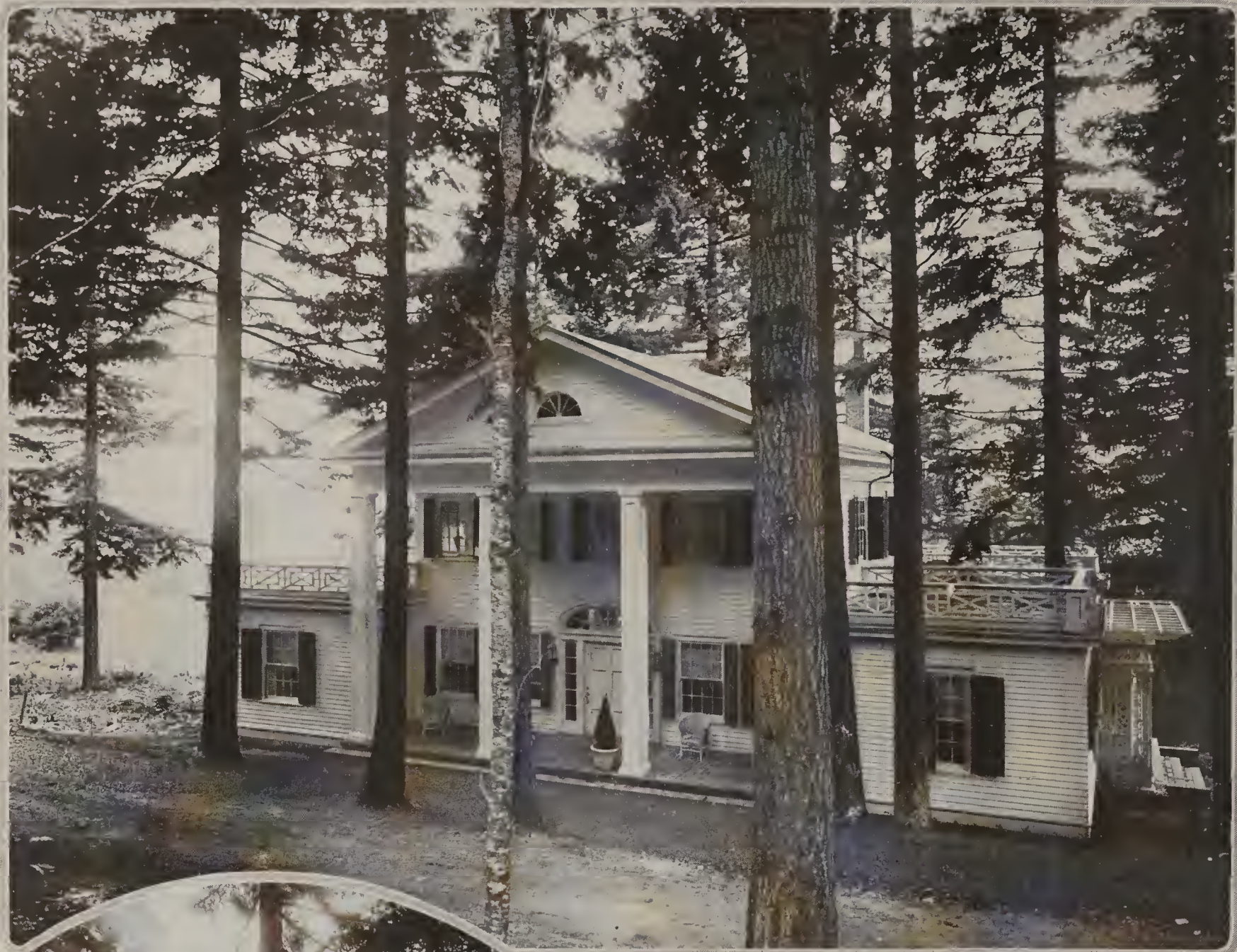
"Forest Hall" stands in a grove of towering firs, the replica of an old Alabama mansion transplanted to the northwest. From the windows one commands a view of the mighty Columbia River, two hundred feet below. The house is clapboard with green blinds
