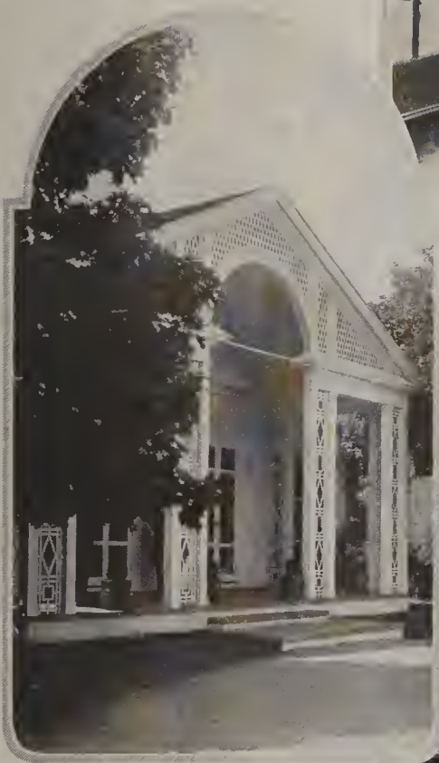
The main entrance is an arched portico supported by delicate trellis panels. Vines which will be trained up these posts will help to complete the picture. From the portico broad flat steps lead down to the drive. This entrance commands a wide stretch of lawn
