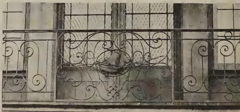
Part of the wrought iron balcony, showing iron ship in full sail; from a warehouse in Philadelphia owned by Stephen Girard and built in 1796
