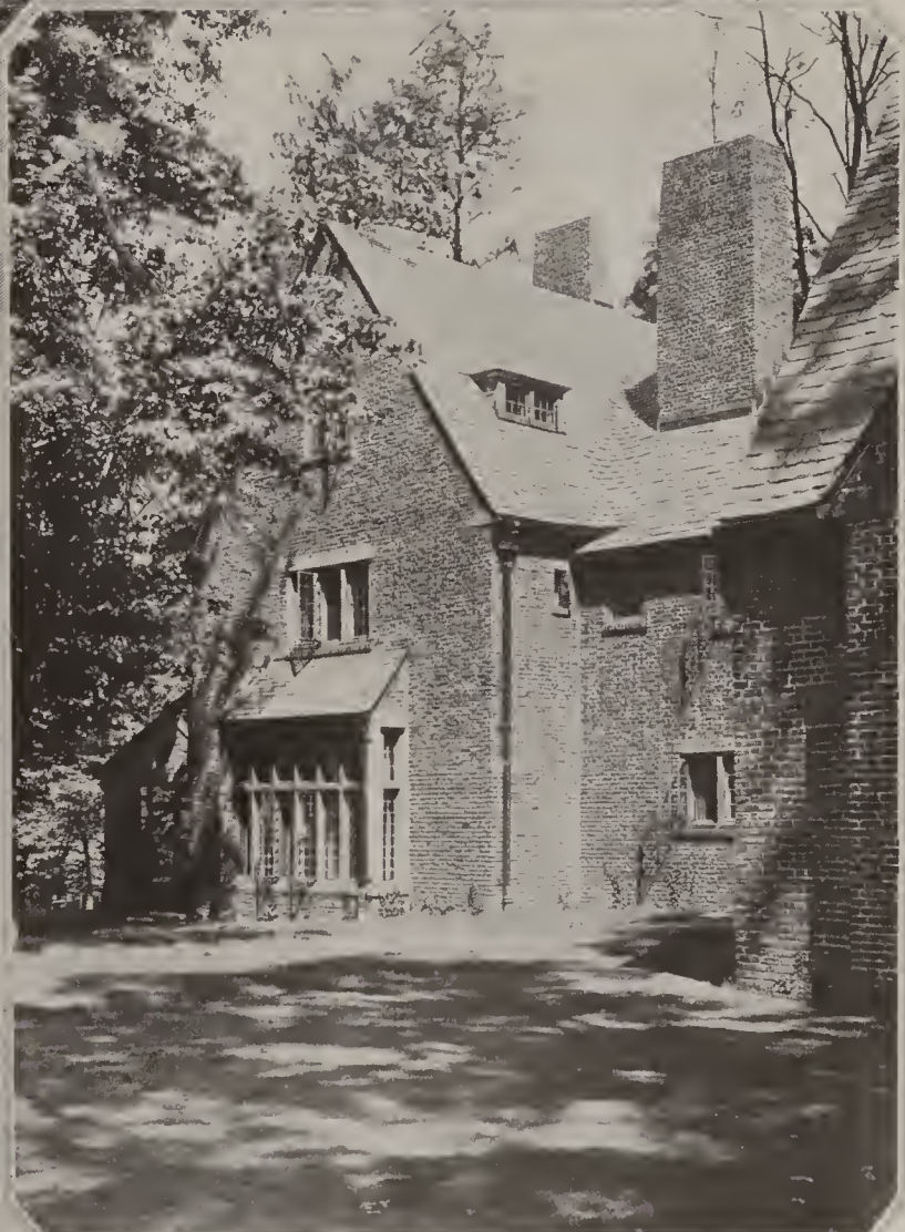
This detail of the exterior shows the uneven quality of the brick and the unusual disposition of the casements that give the façade character
