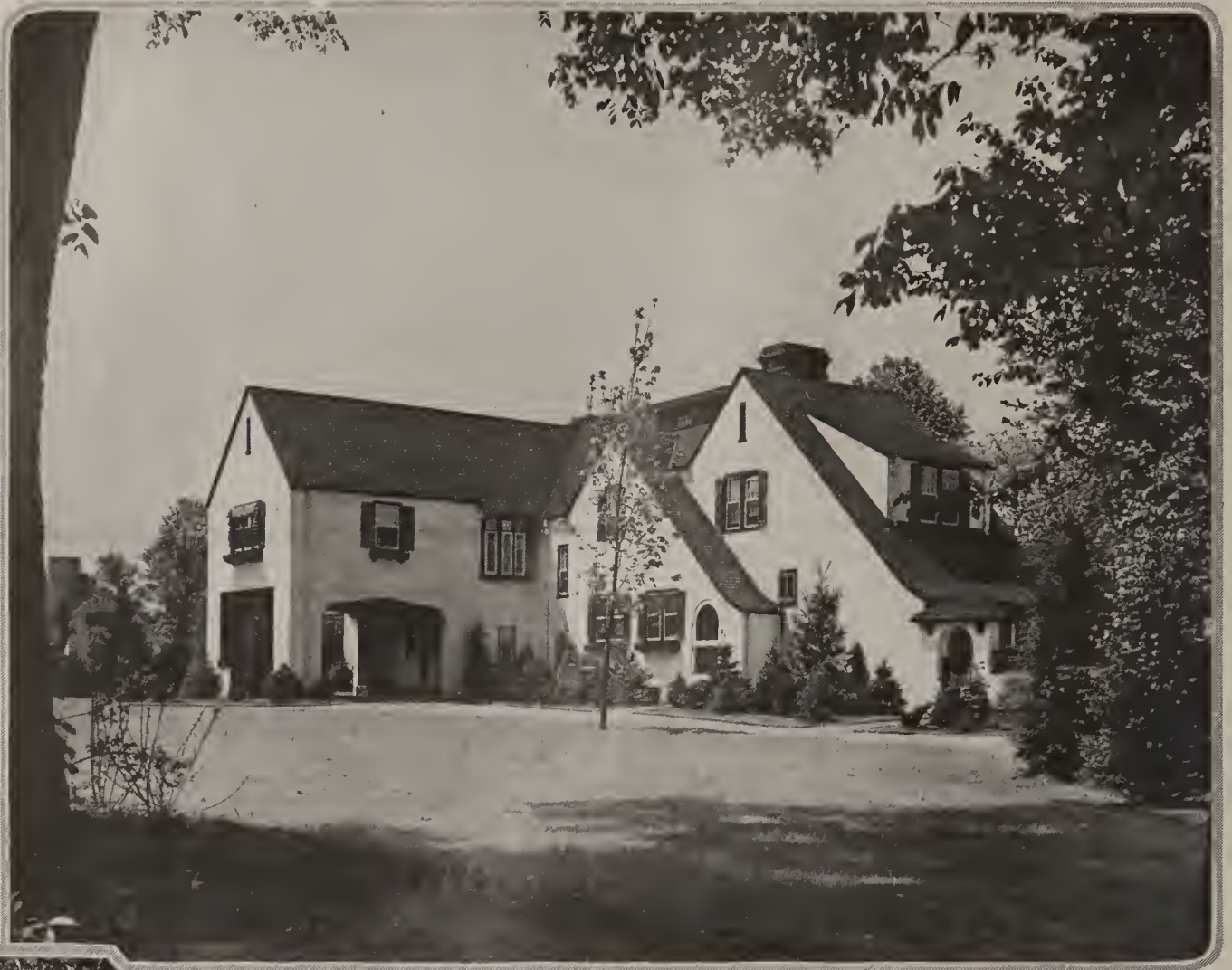
Broken and repeated roof lines give the house unusual architectural interest. These together with the grouping of windows and the arched gate and door, and the oriel up under the eaves of the ell, produce a pleasing façade full of contrasts and rich in texture
