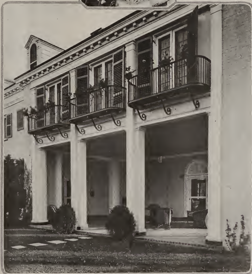
Wrought iron balconies with brackets beneath are used above the sun porch of the Francis L. Hine residence at Lattington Road, L. I. Walker & Gillette, architects
