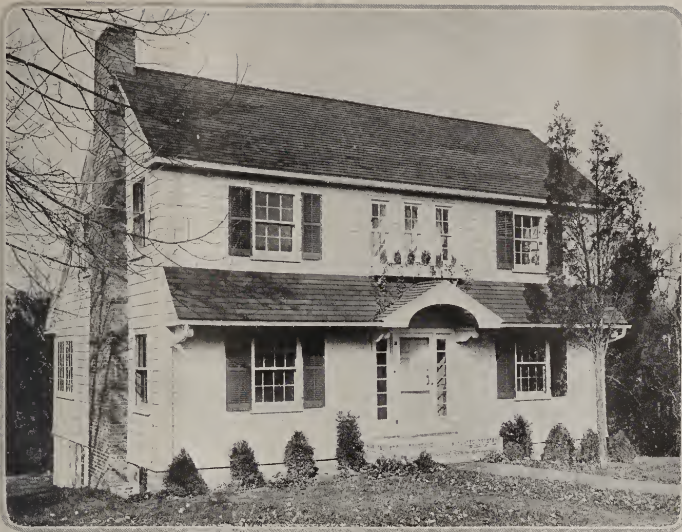
Colonial characteristics adapt themselves readily to the small house. In this little cottage a Germantown hood marks the entrance and the continued pent roof breaks the façade pleasantly. Wide red cedar shingles have been used to cover the exterior walls. They are laid 11" to the weather and painted white. The roof is of similar shingles stained moss green
