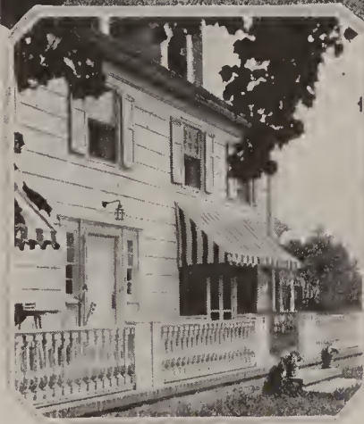
Along the front was built a brick terrace with a balustrade and step leading down to the lawn
