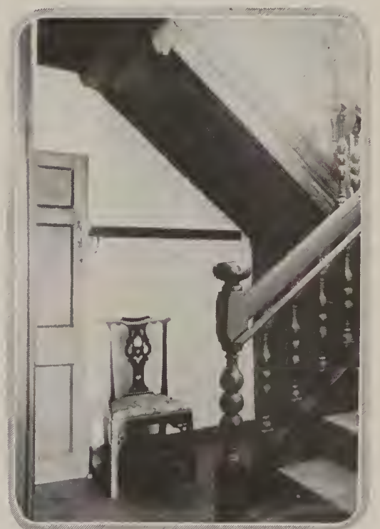
Late 17th Century type of double-bellied spindles and turned newel. "Norwood," Bermuda
