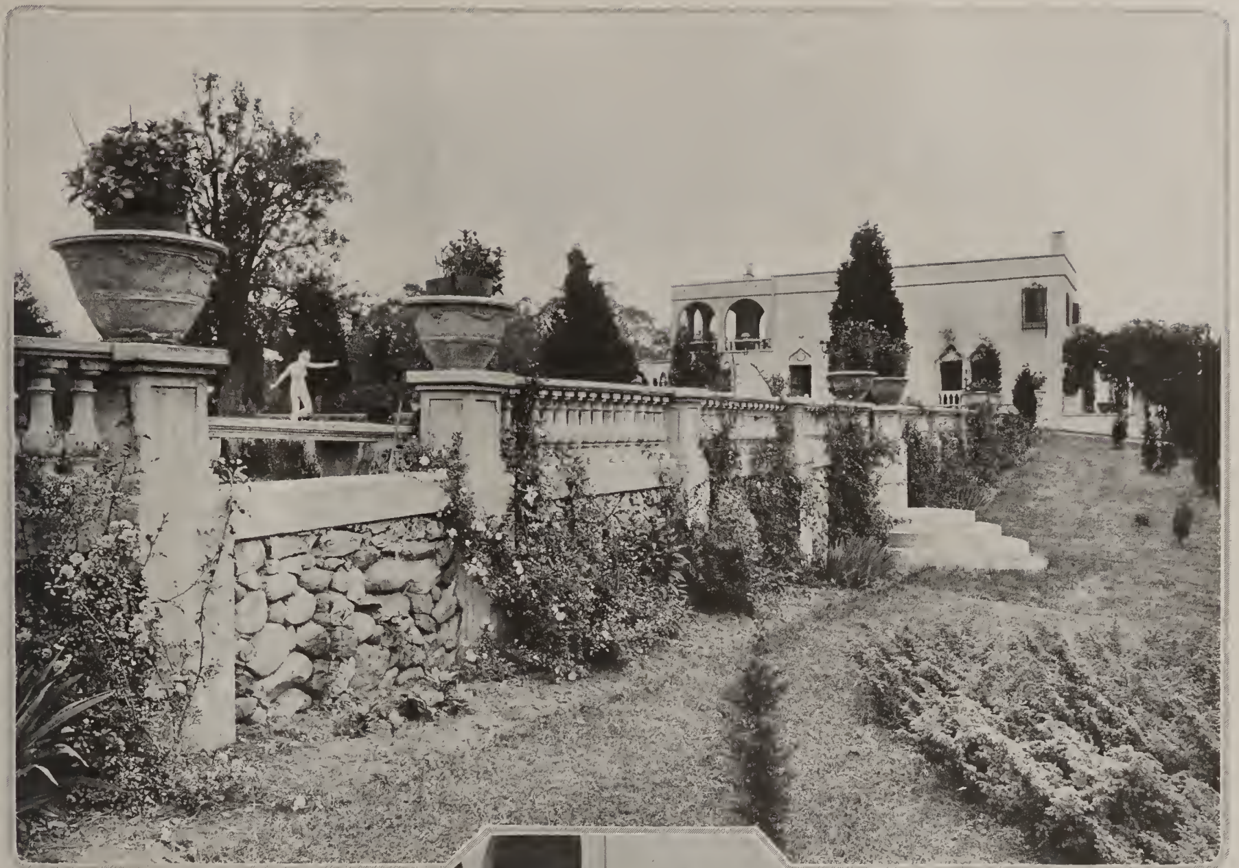
In front lies an Italian garden with a dignified balustrade capping the rubble wall and accented by heavy cement flower jars. Steps lead down to the lawn from the cross axis of the garden
