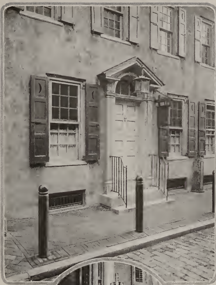
Wrought iron handrails to the doorstep of the Franklin Inn Club, Philadelphia
