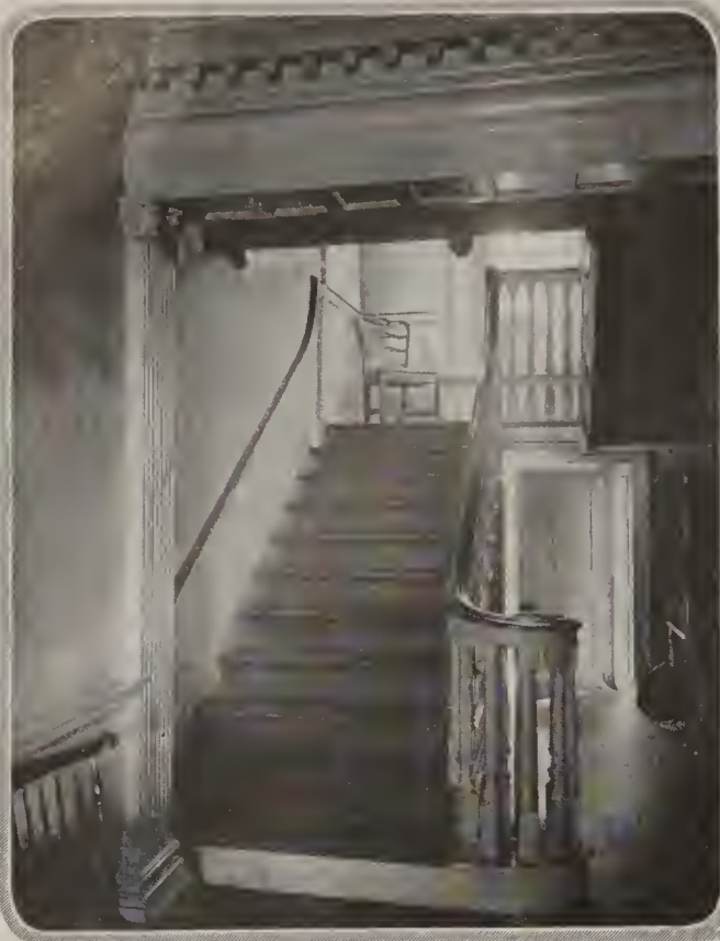
An excellent example of a whorl newel—a small turned newel encircled by a whorl of spindles—is found in "Whitby Hall," Philadelphia
