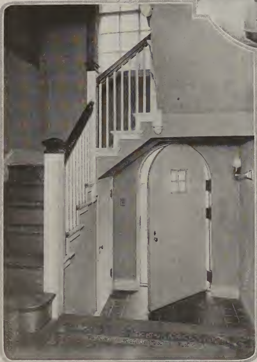
Square spindles and newels with mahogany hand-rails and cap constitute a good modern usage. E. B. Gilchrist, architect
