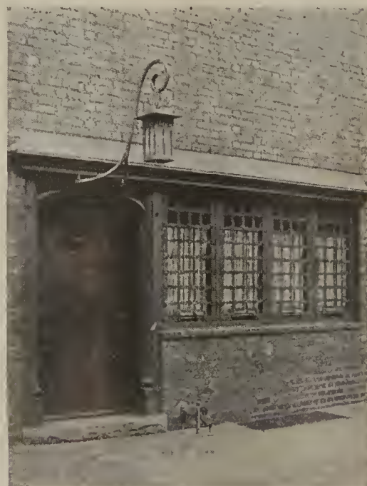
Wrought iron window grill, showing adaptation of Italian inspiration to modern needs. Mellor & Meigs, architects
