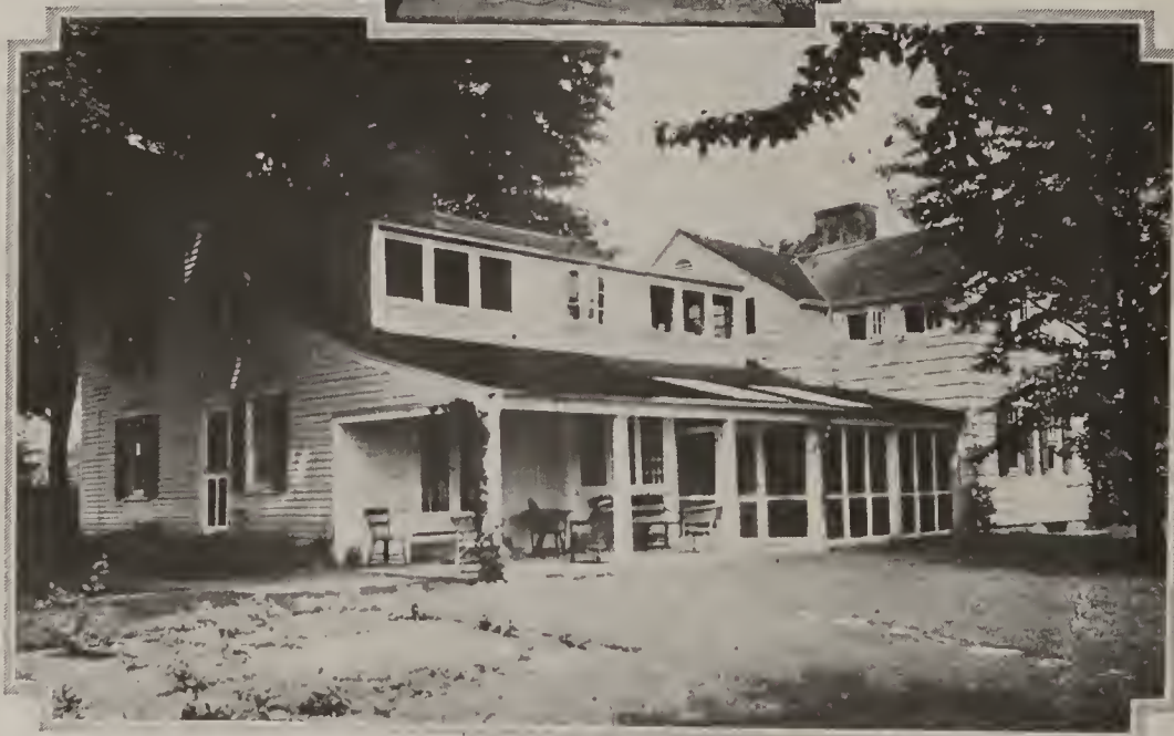
The roof swings low in the rear, covering a broad porch. A long dormer adequately lights the upstairs chambers
