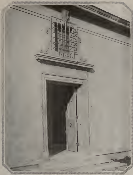
The sharp contrast between this Spanish Renaissance iron window grill and the stucco surface of the wall gives the whole composition a remarkable touch of piquancy. Mellor & Meigs, architects
