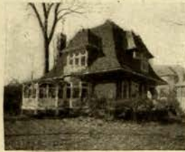
A No. C-241 IDEAL Boiler and 555 ft. of 38-in. AMERICAN Radiators, costing the owner $250, were used to Hot-Water heat this cottage.
