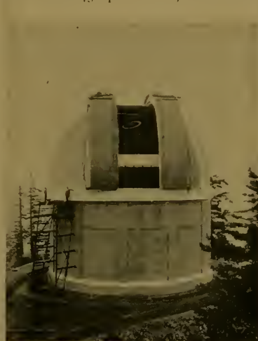
FIG. 4.—The Observatory, October 22, 1916. The shutters are open their full width (15 ft.), and the wind-shield is seen before the telescope.
