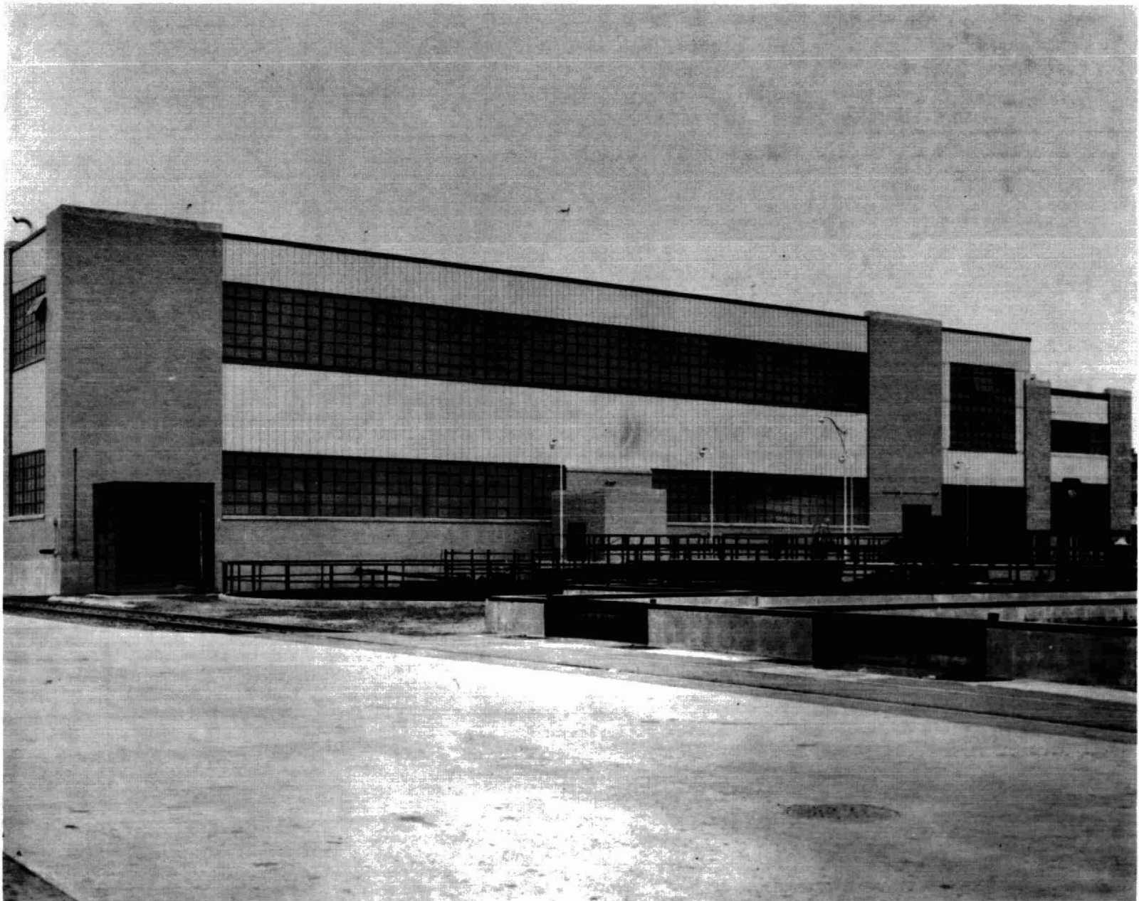
— FIGURE 8, CONTROL BUILDING FOR LARGE OIL WASTE TREATMENT PLANT —
