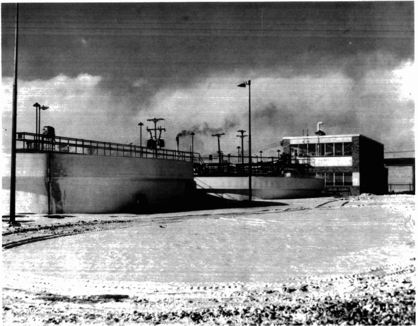
— FIGURE 9, LARGE OIL WASTE AND PLATING WASTE TREATMENT PLANT HANDLING 1900 GALLONS PER MINUTE STORM SEWER FLOW.
