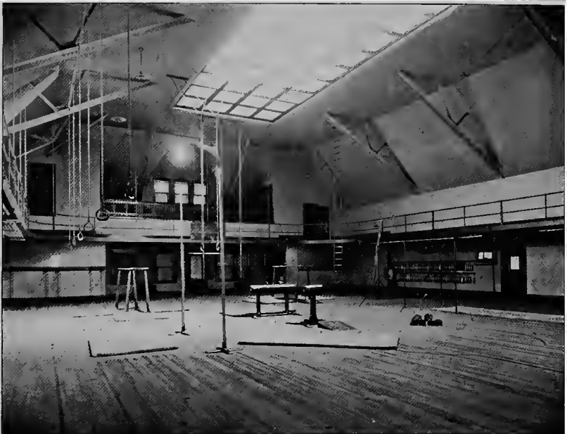
Carnegie library, Homestead: gymnasium, showing suspended running track
