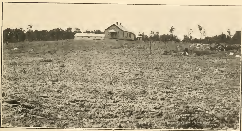
FIG. 2. VIEW OF NEWLY CLEARED FIELD ON COLOMA LOAM AT GOODMAN.
