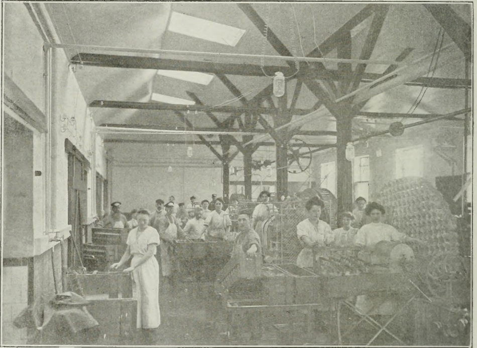
Interior of Copenhagen Dairy.
