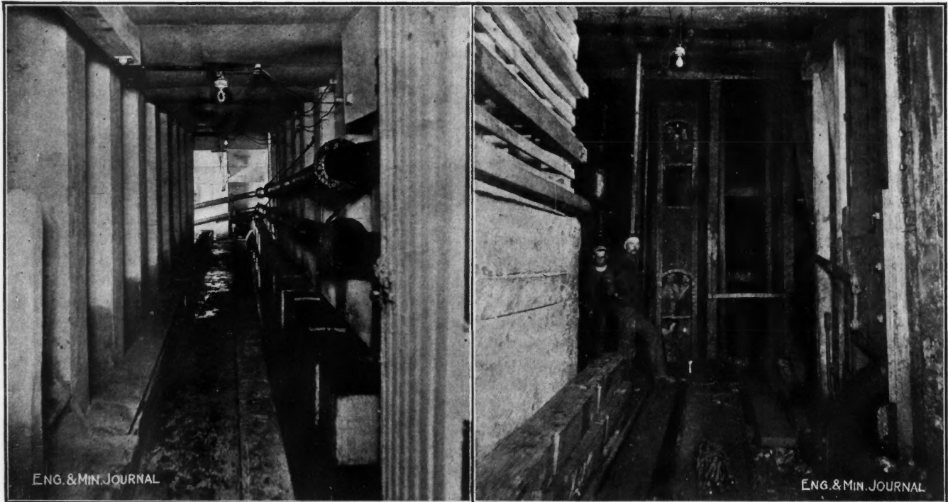
Entrance to electric-pump chamber and sump at 2430-ft. level
