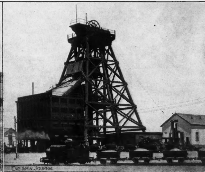
HEADFRAME AND ORE BINS AT TAYLOR'S SHAFT
