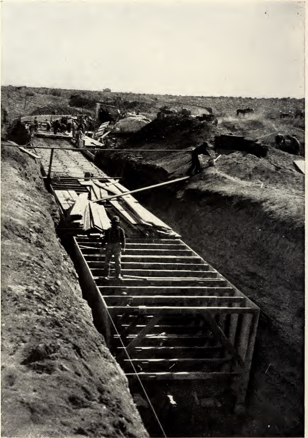
PLACING THE FORMS, TO BE FOLLOWED BY THE POURING OF CONCRETE
