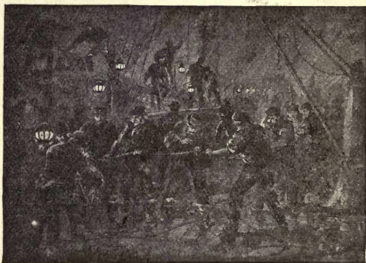
FIG. 39.—“Foul in tank” whilst paying-out.
