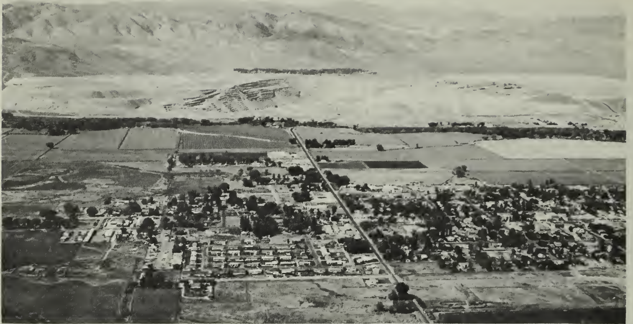
Anaconda Copper Corp. Weed Heights operation near Yerington is the center of Basin mineral industry, Walker Subbasin
