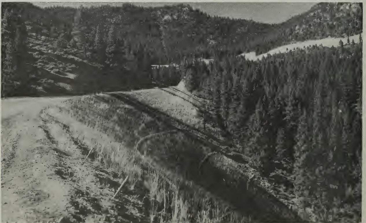
This seeded and treated highway fill in the Carson Subbasin will reduce sediment production and erosion. Forest Service photo.
