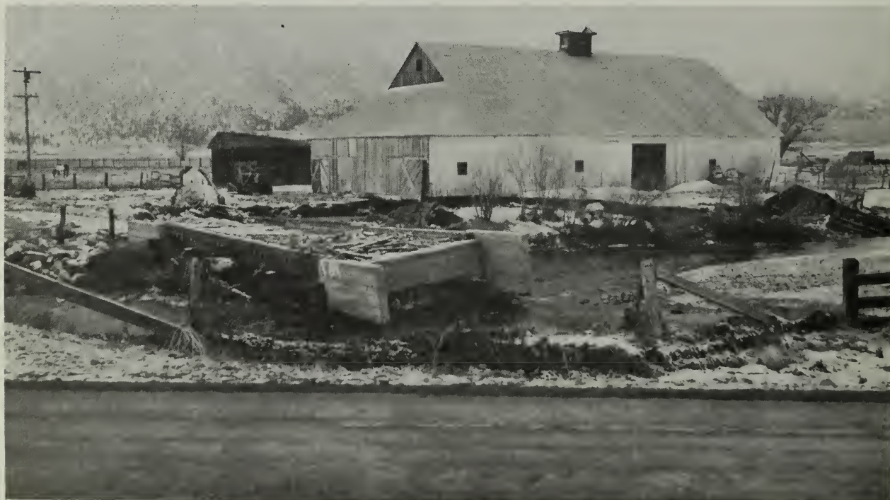
Flood damage from West Fork Carson River, Carson Subbasin.
