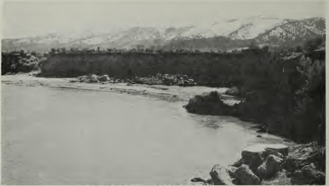
The upper Long Valley watershed, Calvada Subbasin, presents severe streambank erosion problems.
