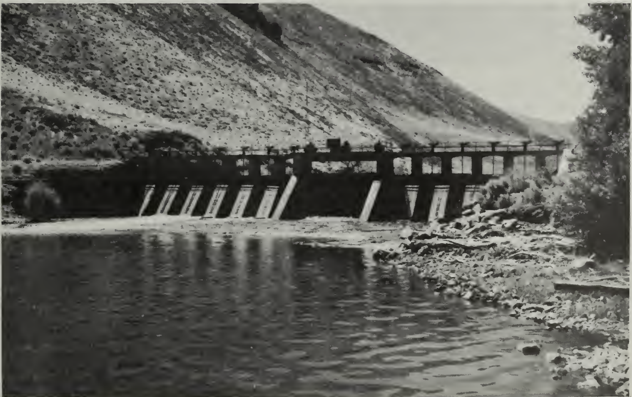
Derby diversion dam on the Truckee River diverts water to Lahontan Reservoir for use in the Carson Subbasin.
