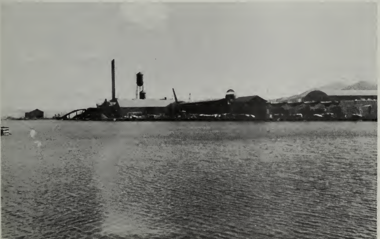
Wood products processing plant at Susanville, Calvada Sub-basin. The Subbasin is the center of the Basin's wood products industry.
