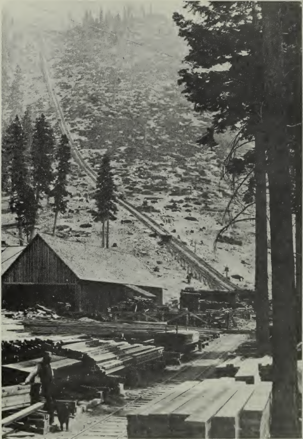
Inclined railway of the Sierra Nevada Wood & Lumber Company at Incline Village, Lake Tahoe, about 1890. Finished lumber was hauled to the top of the incline, then transported by V-flume to Carson City and hauled by rail to Virginia City. The denuded slope in the background was typical of the Sierra Nevada timberlands after logging. The Ponderosa Ranch recreation facility now stands on this site. Victor Goodwin photo.
