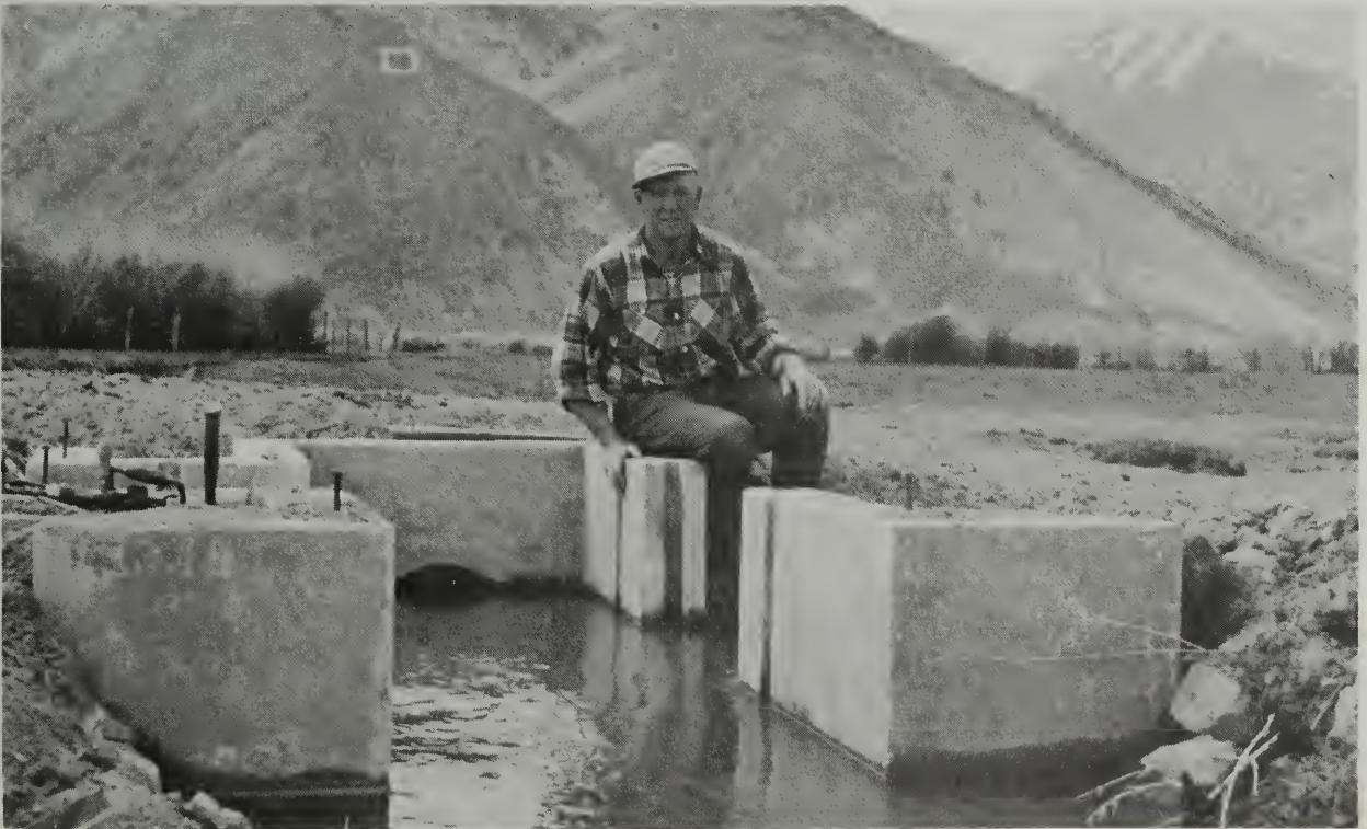
Concrete irrigation water control structures are an important element under the USDA Public Law 46 program.
