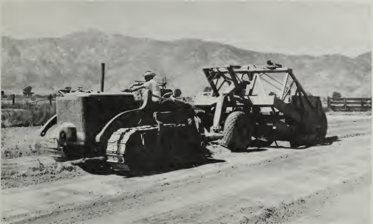
Many thousands of acres of the Basin irrigated croplands have been levelled to provide a uniform grade for irrigation
