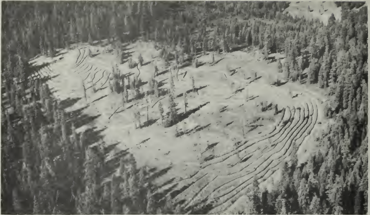
Because of pressures to remove pollutants from the Lake Tahoe Basin, a "cinder cone" is utilized for disposal of primary settled sewage effluent. About 15,000 feet of trenches are used to permit settlement and percolation.
