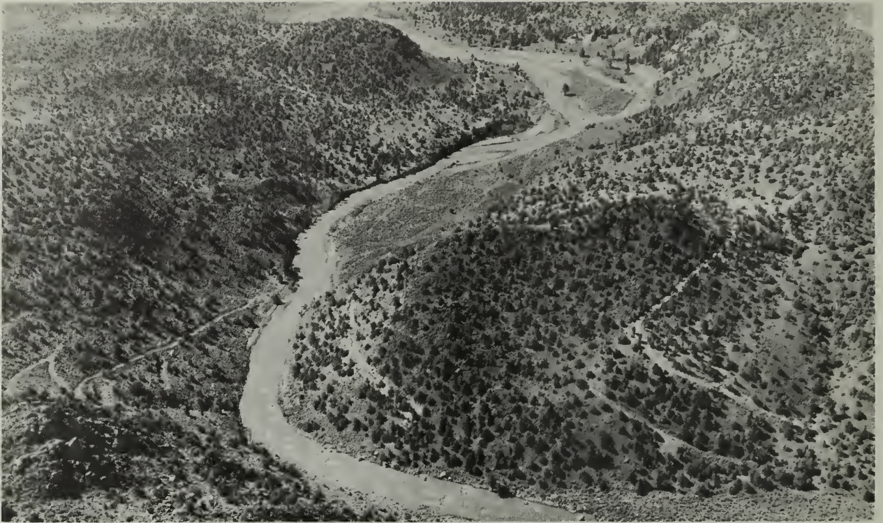
Watasheamu dams site on the East Carson River, a major feature of the U. S. Bureau of Reclamation Washoe Project.
