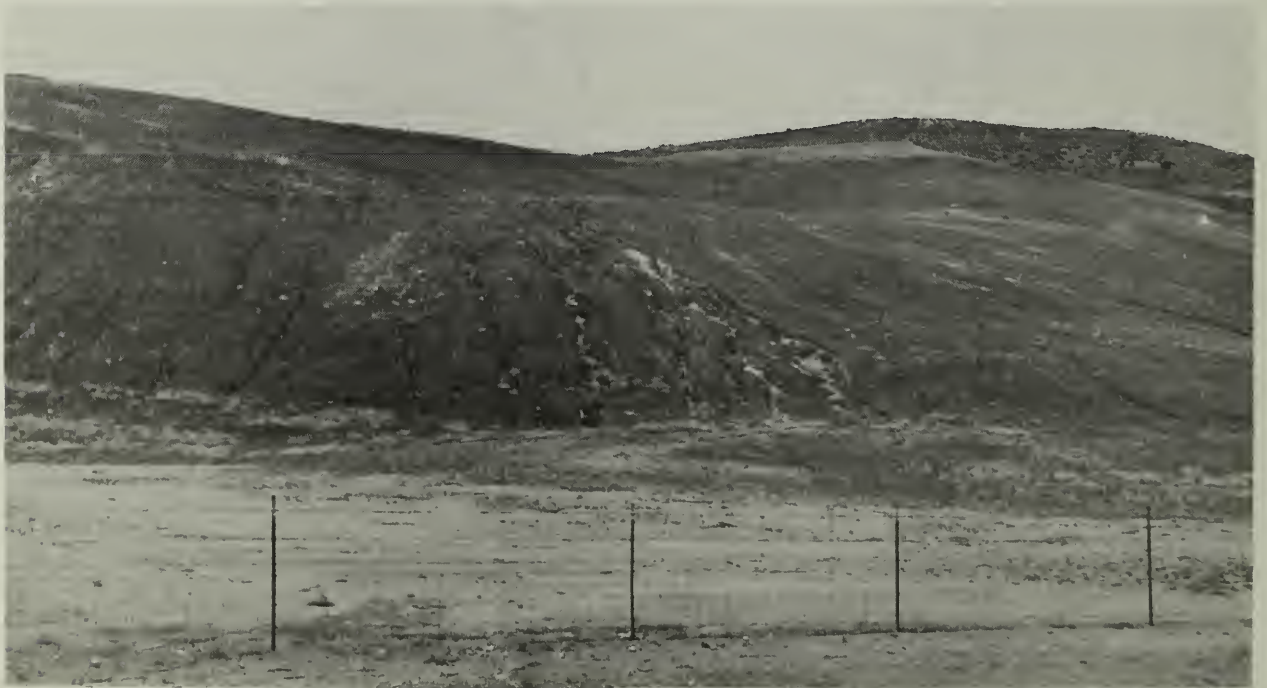
This borrow pit, which resulted from freeway construction, has been smoothed and seeded by Nevada Highway Department to reduce erosion and sedimentation. Truckee Subbasin
