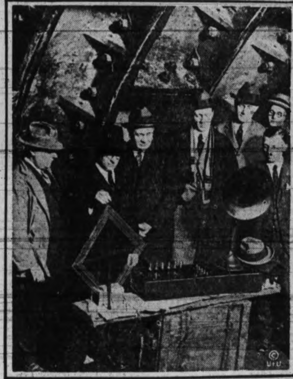
YOU CAN'T KEEP THEM OUT! —Radio waves will penetrate just about everything! A test was made recently 90 feet below the surface of the Hudson River at New York City, in the steel tube of the new tunnel now under construction. Almost perfect reception was recorded. Major Gleim (extreme left) is chief engineer of the new tunnel, an engineering marvel.
