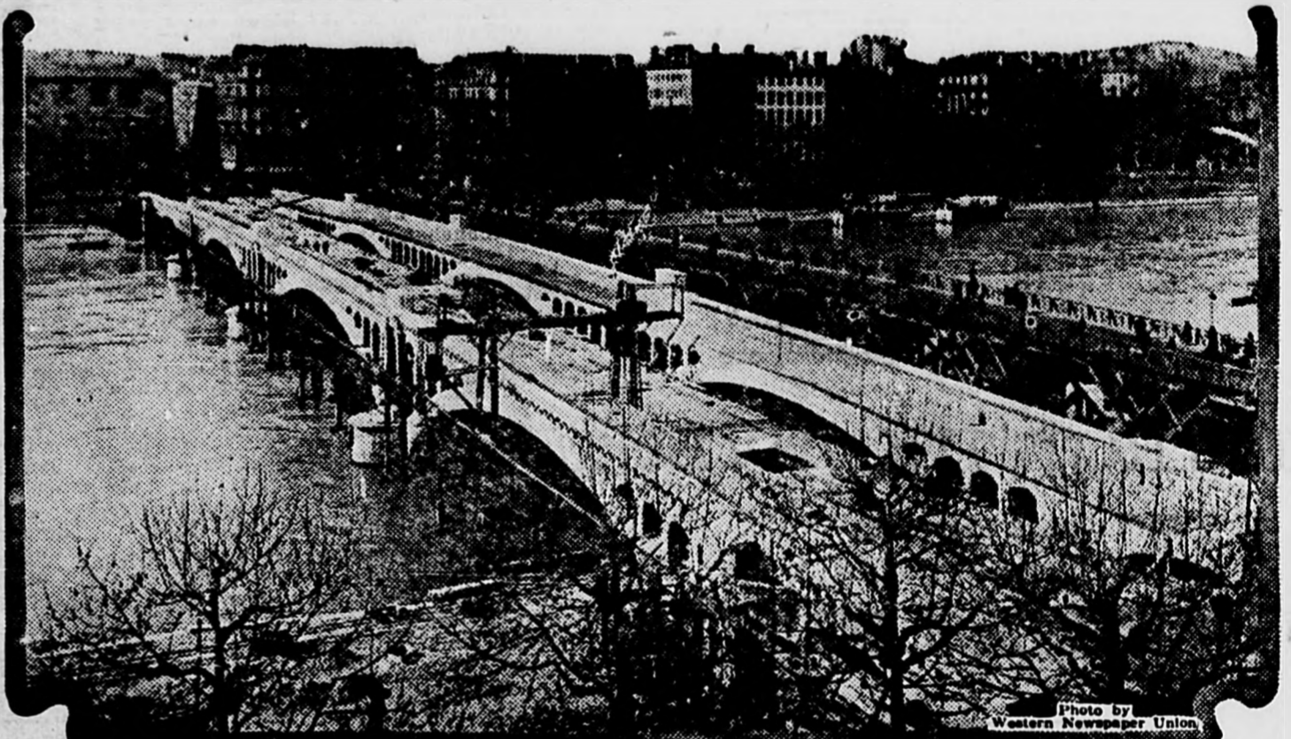
This is the new President Wilson bridge across the Rhone at Lyons, France, which has just been dedicated. It was begun since the starting of the war.
