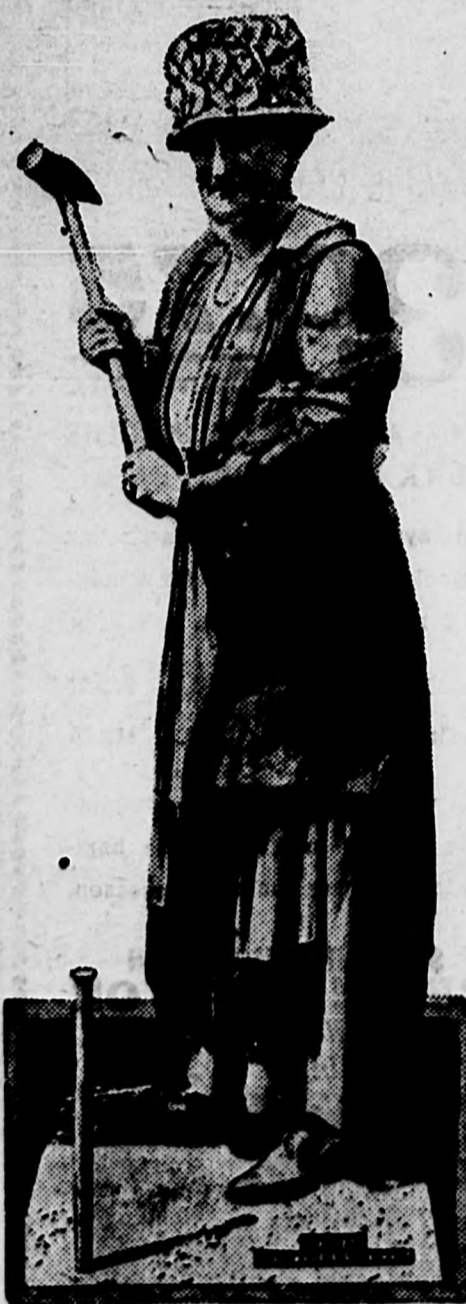
Prominent Y. W. C. A. workers who were holding a convention in Portland, Me., visited a shipyard where the trawler Albatross was under construction. Mrs. John D. Rockefeller, Jr., tried her hand at driving a bolt in the keel, and wielded the hammer with skill and force.
