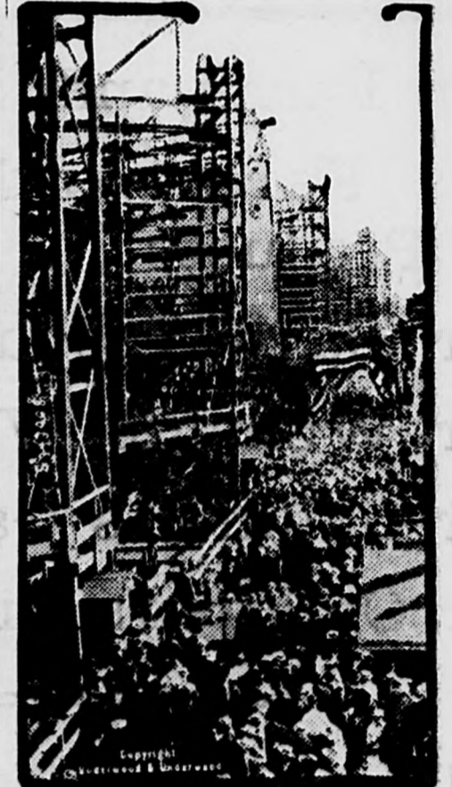
View of the shipways at Newark Bay yards as the Alamosa, Alcona and Chetopa were launched simultaneously.
