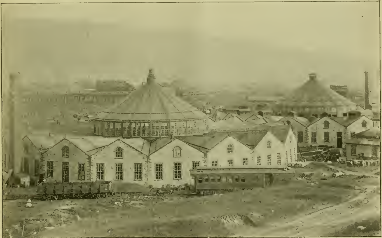
ROUNDHOUSE OF THE PHILADELPHIA & READING RAILROAD AT READING, PA., BUILT IN 1865.
