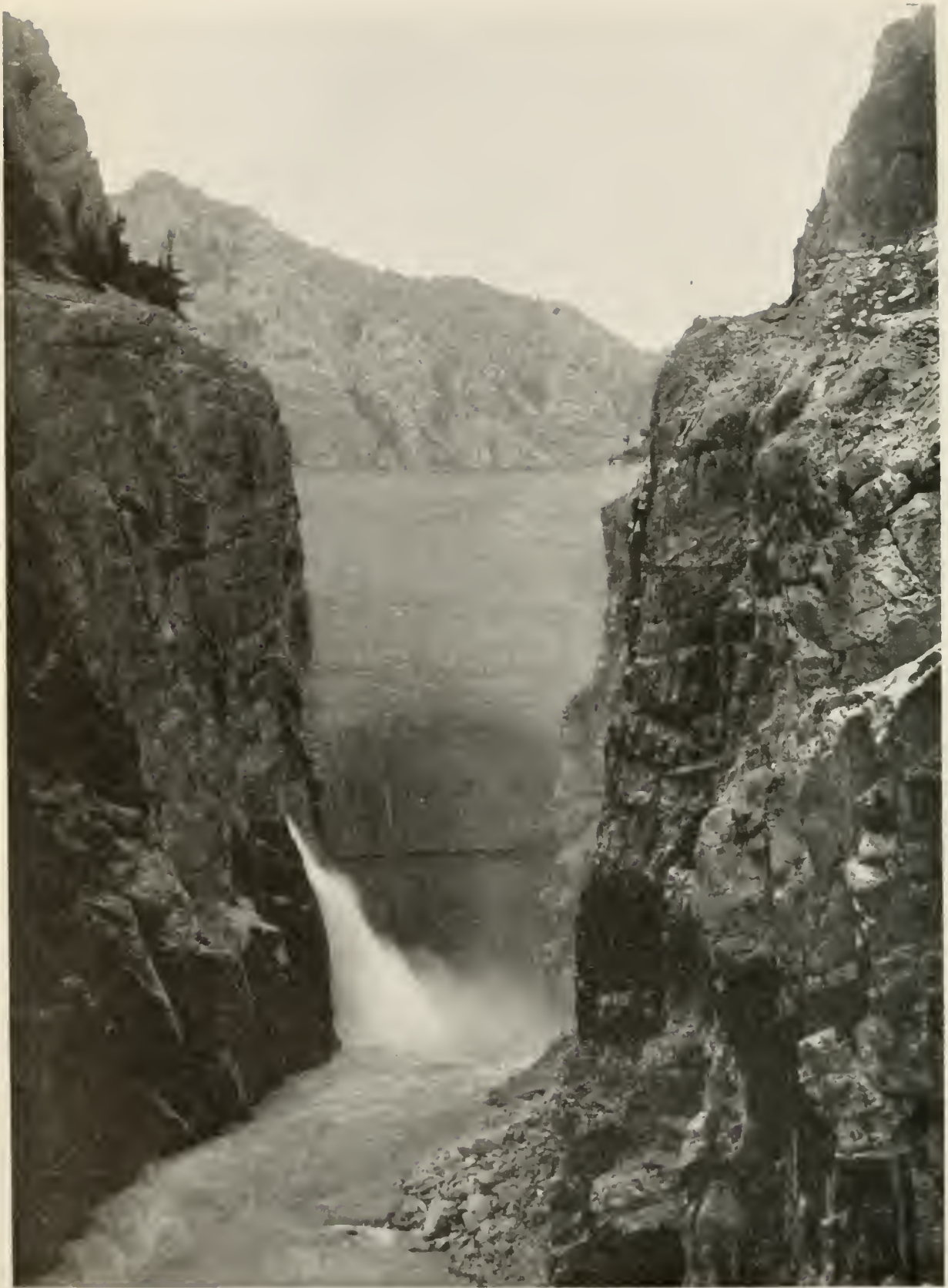
SHOSHONE DAM WYOMING, 328.4 FEET HIGH. HIGHEST DAM IN THE WORLD. 80 FEET LONG AT BOTTOM, 200 FEET AT TOP.
