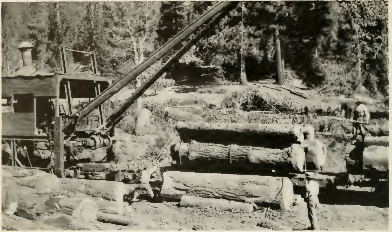
STEAM LOADER ON MARCH LUMBER COMPANY'S LOGGING RAILROAD, PLUMAS NATIONAL FOREST.
