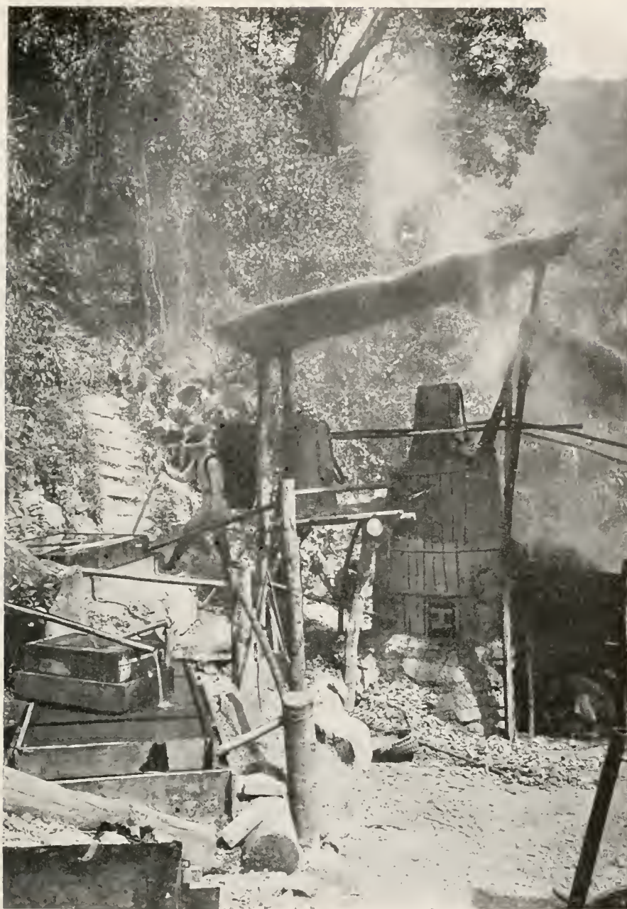
A TYPE OF ONE OF THE MANY CAMPHOR MANUFACTURING KILNS WHICH ARE FOUND IN THE FORESTS OF FORMOSA.
