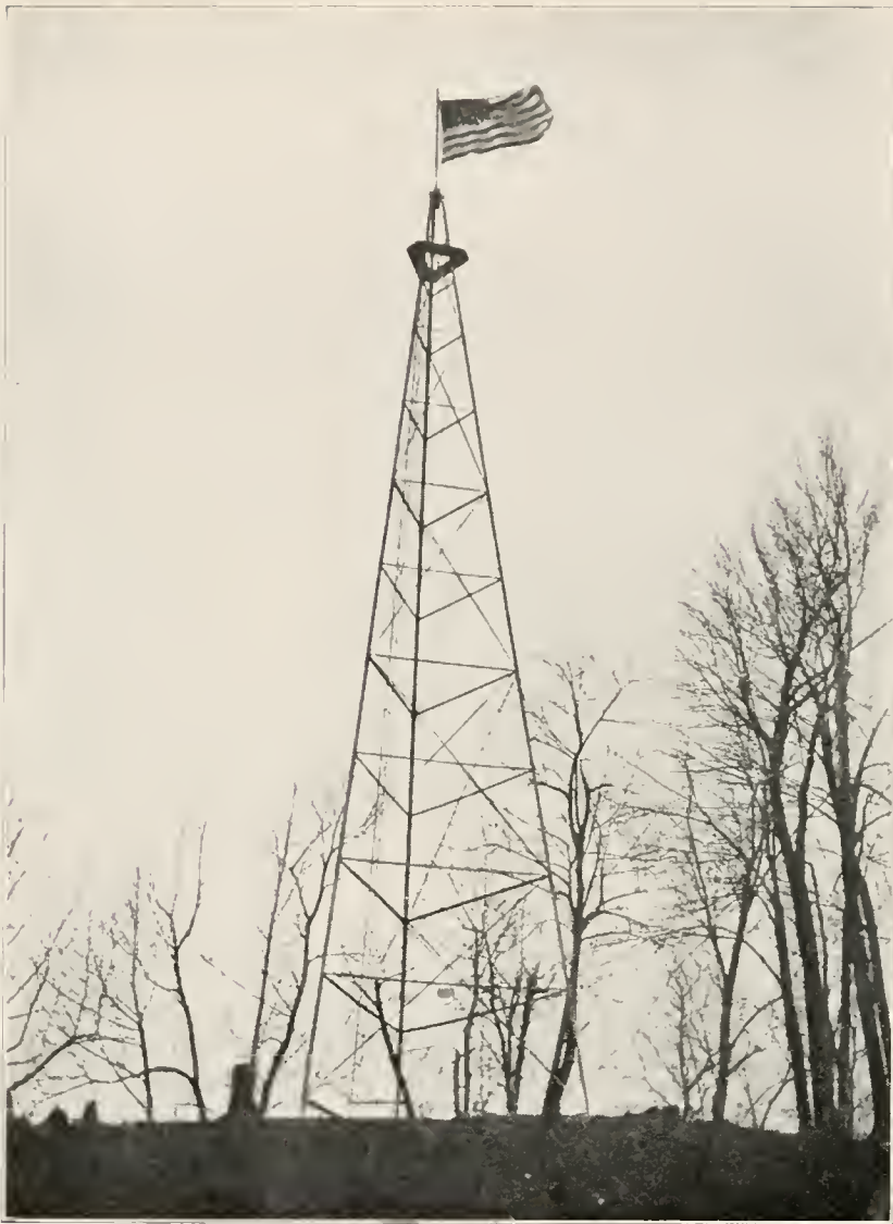
MINNESOTA FOREST SERVICE STEEL TOWER AT GULL LAKE, ERECTED AUGUST 25, 1911. COST $36.30.
