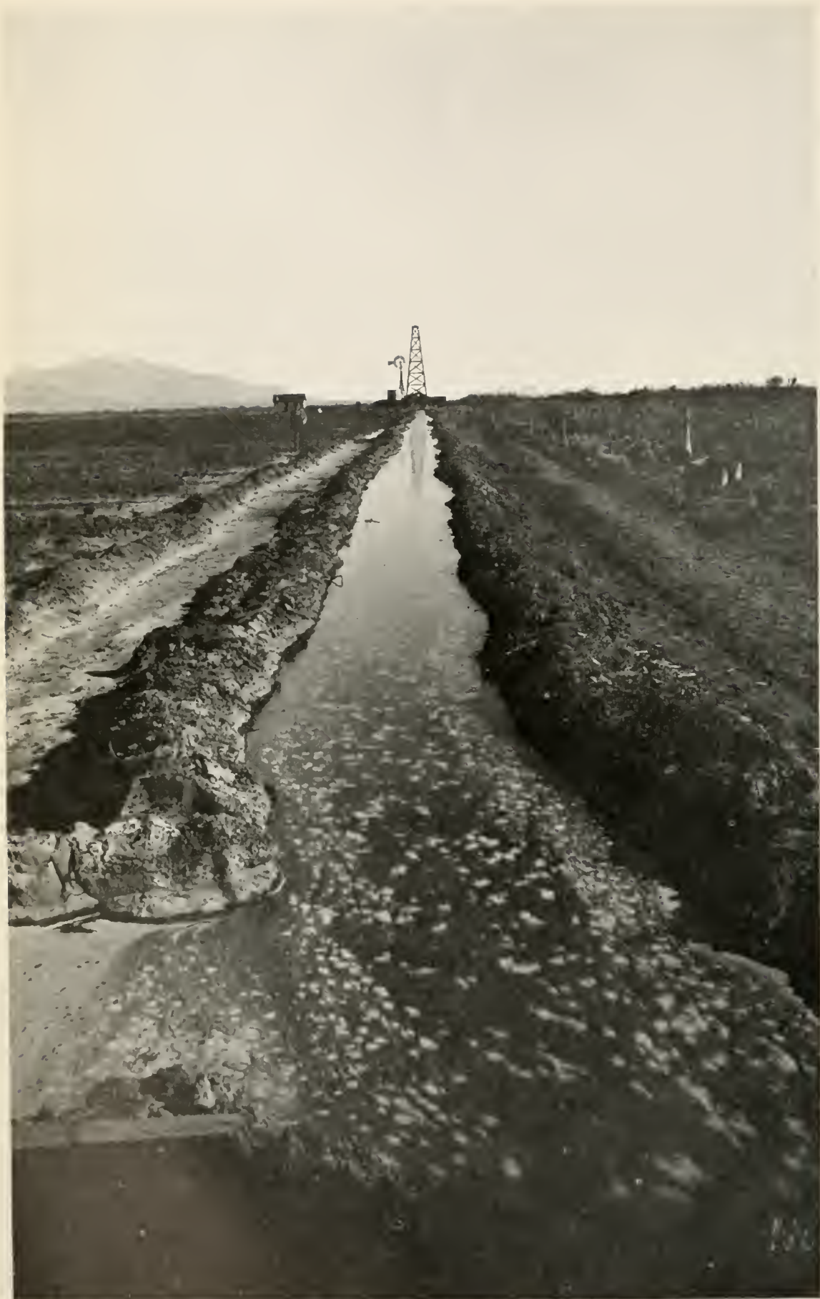
IRRIGATION DITCH SUPPLIED BY WELL PUMPING 1,300 GALLONS OF WATER PER MINUTE NEAR DEMING, N. M.
