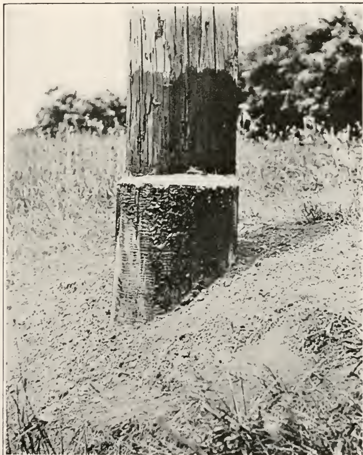
FINISHED POLE ON SLOPE.
