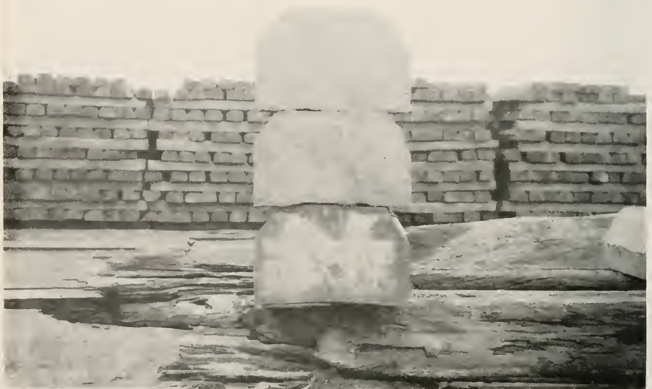
CROSS SECTIONS OF BEECH TIE TREATED BY THE REUPING PROCESS AT STENDAL, GERMANY.
