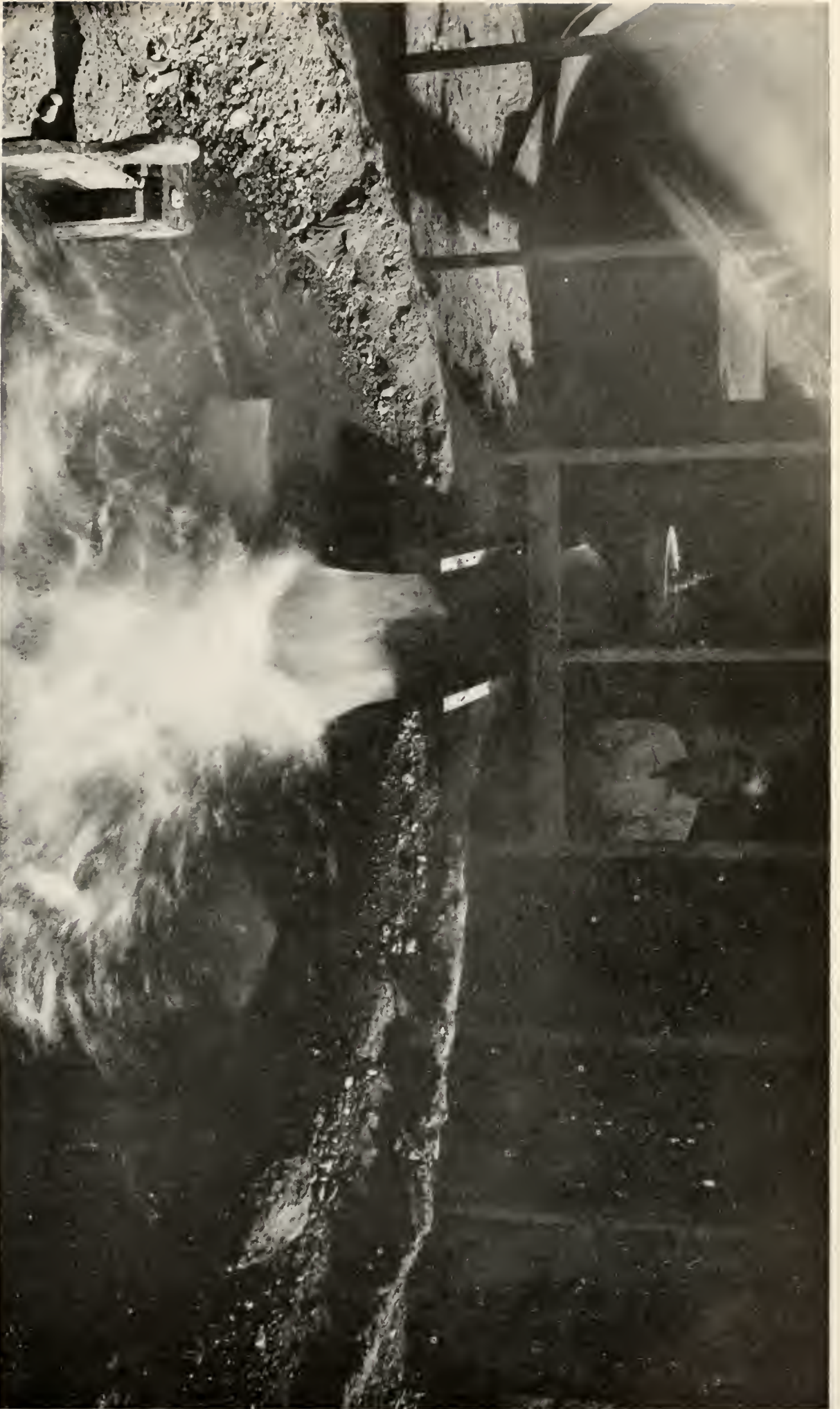
WELL PUMPING 1,400 GALLONS PER MINUTE FOR IRRIGATION FOUR MILES EAST OF DEMING, N. M.
