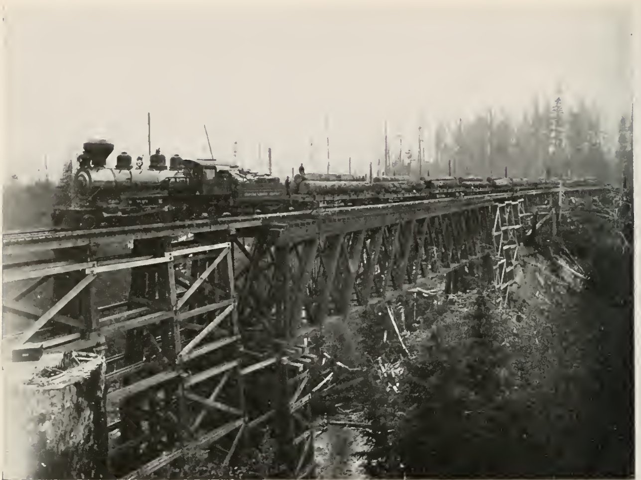
BRIDGE OVER WEST FORK OF TATSOP RIVER, 130 FEET ABOVE THE RIVER. WITHIN ONE MILE ON THIS SAME ROAD IS THE TWIN OF THE BRIDGE. IT IS ESTIMATED THAT THE LAST 1\frac{1}{2} MILES OF THIS ROAD, INCLUDING THESE BRIDGES, COST NEARLY $100,000 TO PUT INTO OPERATION. IT IS STRICTLY A LOGGING ROAD. SIMPSON LOGGING CO., SHELTON, WASH.
