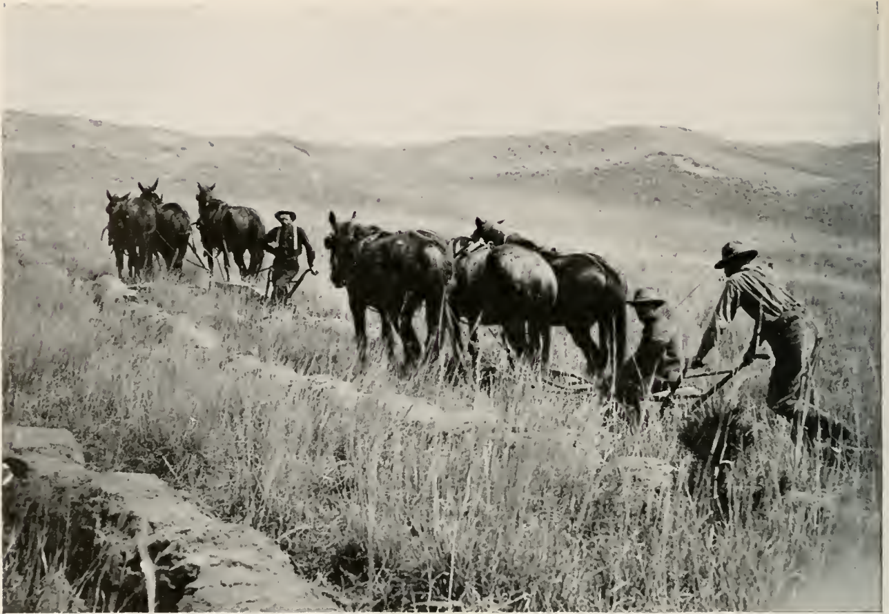
THE PLOW WITH TRENCHER FOLLOWING
