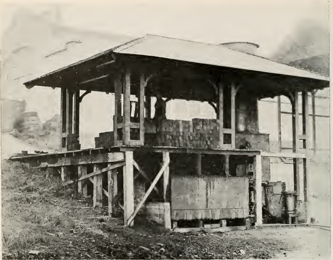
OPEN TANK PRESERVATION PLANT
