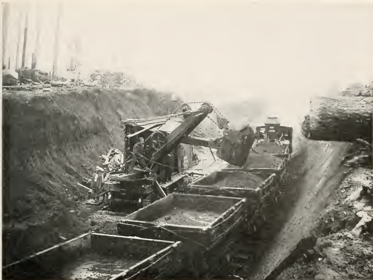
STEAM SHOVEL AT WORK ON NEW EXTENSION, SIMPSON LOGGING CO.'S R. R. AT SHELTON, WASH. CONSTRUCTION OUTFIT OWNED AND OPERATED BY THE LOGGING COMPANY.
