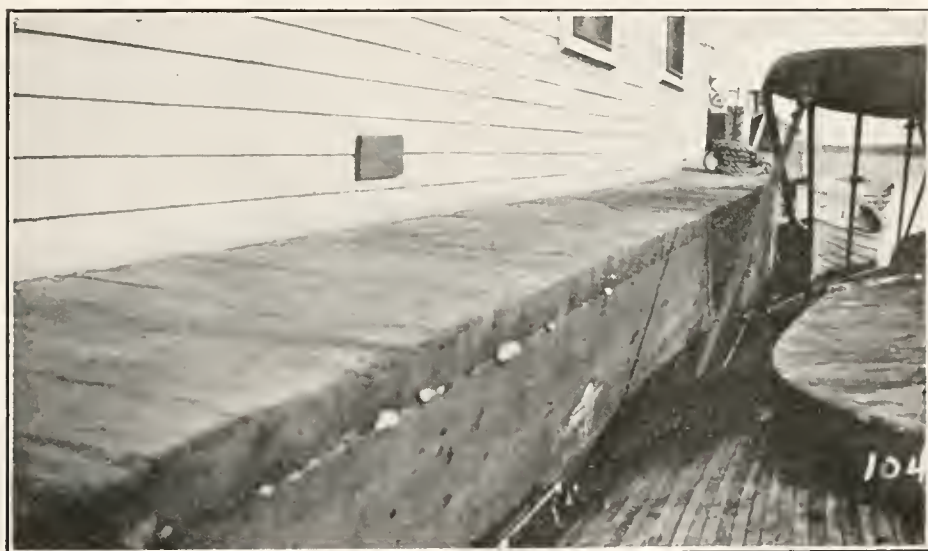
UNTREATED DOUGLAS FIR HULL, FOUR YEARS OLD.
