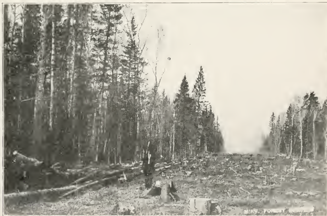
CLEARING RIGHT OF WAY FOR RAILROAD THROUGH DENSE TIMBER—SLASH BURNED CLEAN UNDER DIRECTION OF RANGER—PULP WOOD WILL BE HAULED OFF.
