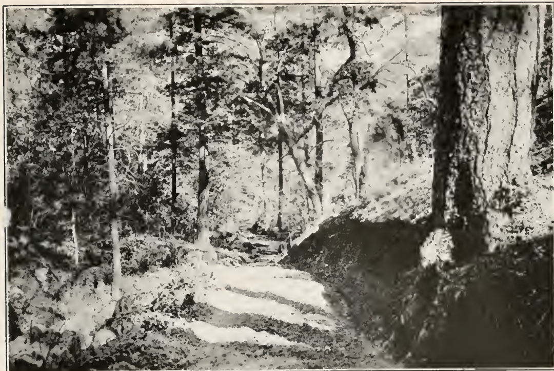
A ROAD ON THE GILA NATIONAL FOREST, NEW MEXICO, WHICH COST $466.00 PER MILE.
