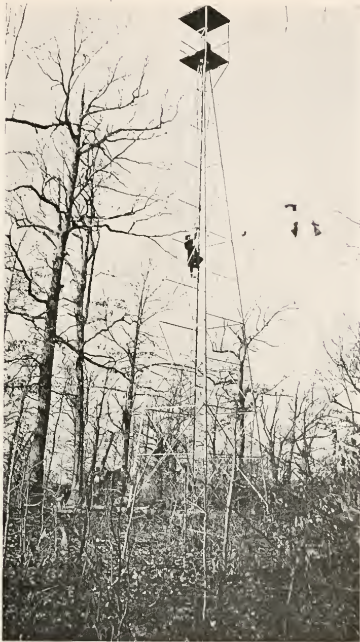
SHOWS LOOKOUT TOWER ON McGOWAN'S POINT. THESE PICTURES SHOW THE NEED OF A HIGH TOWER ON THE OZARK NATIONAL FOREST, BECAUSE OF THE HIGH TREES SURROUNDING. THESE TREES THAT ARE NEAR WILL BE FELLED TO PREVENT DAMAGE BY REASON OF THEIR FALLING AGAINST IT IN A HEAVY WIND STORM. McGOWAN'S POINT, ARKANSAS.
