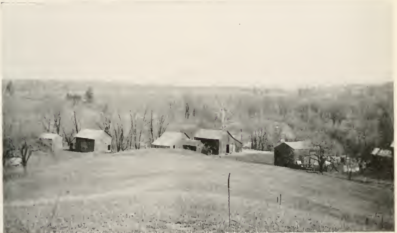
LOOKING OVER LAND THAT WILL BE FLOODED. THE FARM BUILDINGS IN THE PHOTOGRAPH WILL BE TORN DOWN AND REMOVED BECAUSE THEY ARE BELOW THE HIGH-WATER LEVEL OF THE PROPOSED RESERVOIR.
