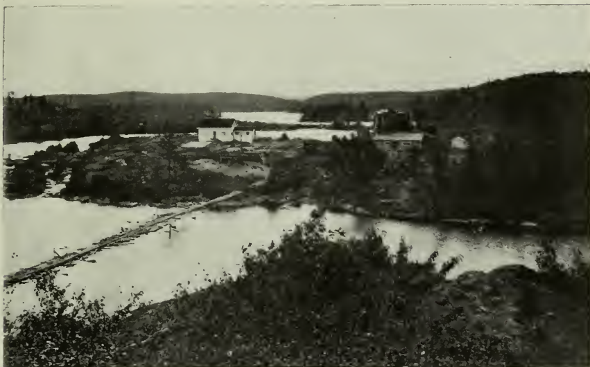
Office and mill, Argonaut gold mine, looking east. Beaverhouse lake is in the distant background, York lake in the foreground.
