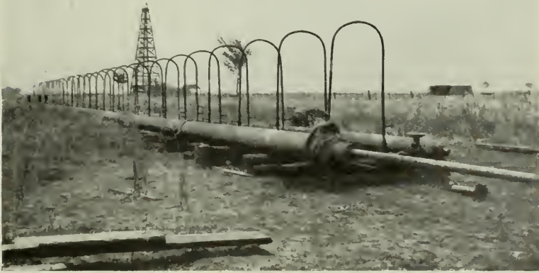
Separator for preventing the oil from a gas well from reaching the gas lines.
