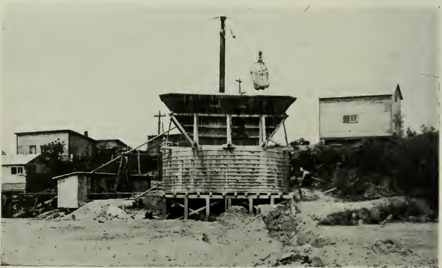
Pioneer drag-line excavator used to reclaim a slime carrying 6 ounces of silver for treatment by the cyanidation process, Coniagas mine. The slime is reclaimed in the moist state, agitated in cyanide solution and pumped to the cyanide plant.
