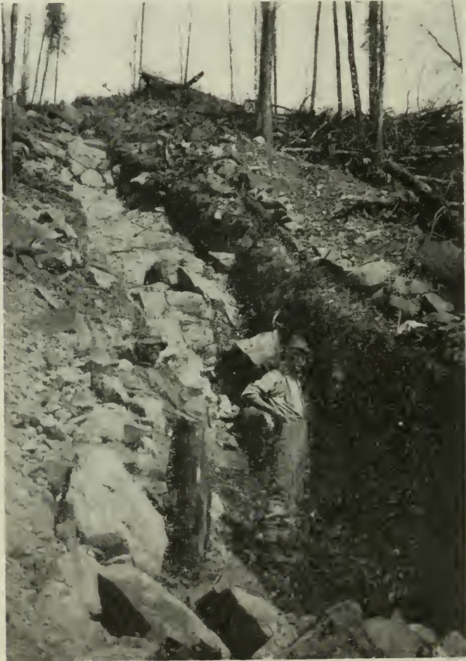
Trenching on claim H.S. 238, at southeast corner of Katrine township.
