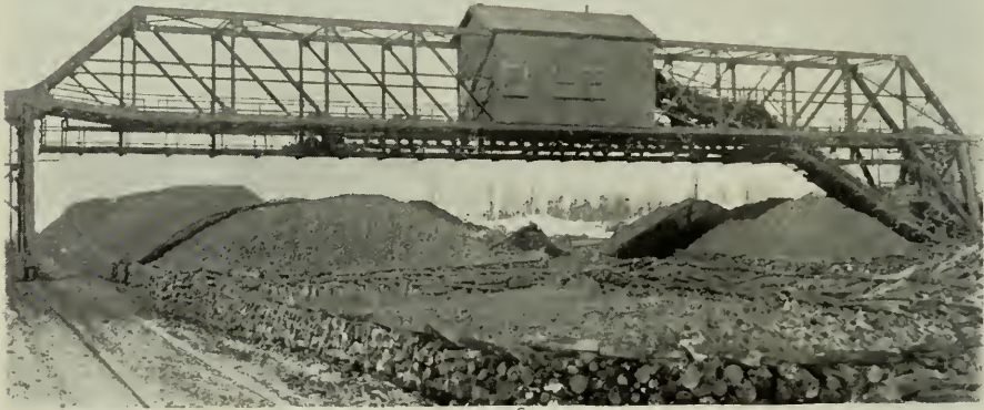
Ore bridge for loading roasting heaps at O'Donnell, International Nickel Company of Canada, Ltd.
