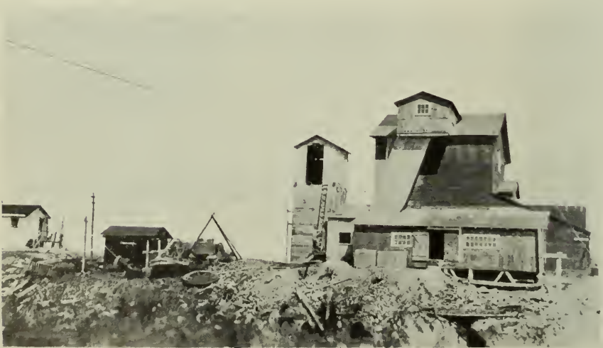
Mill at Argonaut gold mine, township of Gauthier.
