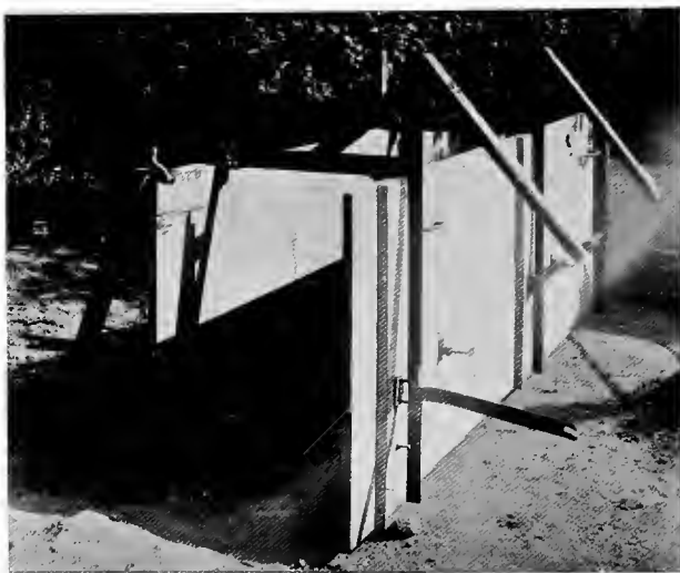
MARK V SHUTTERING.
