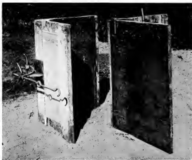
MARK V SHUTTERING,
