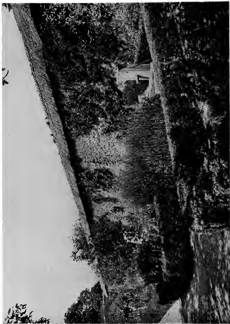
A COB GARDEN-WALL WITH THATCHED COPING.
