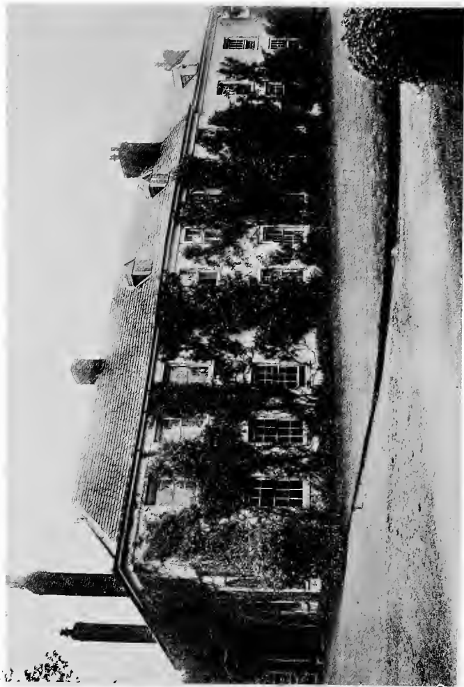
A FINE SPECIMEN OF A DEVONSHIRE COB HOUSE.
