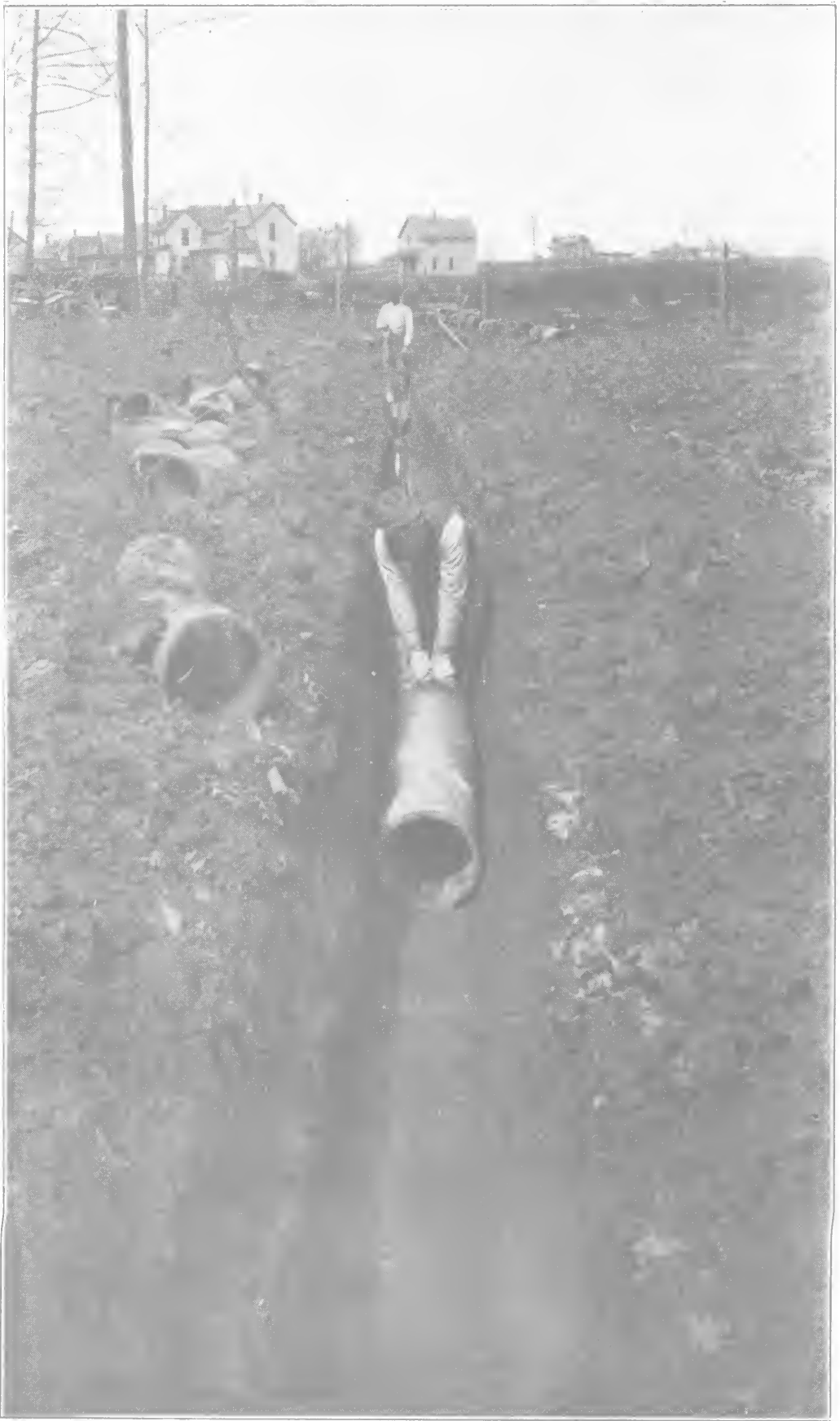
LAYING TWELVE-INCH DRAIN-TILE.
