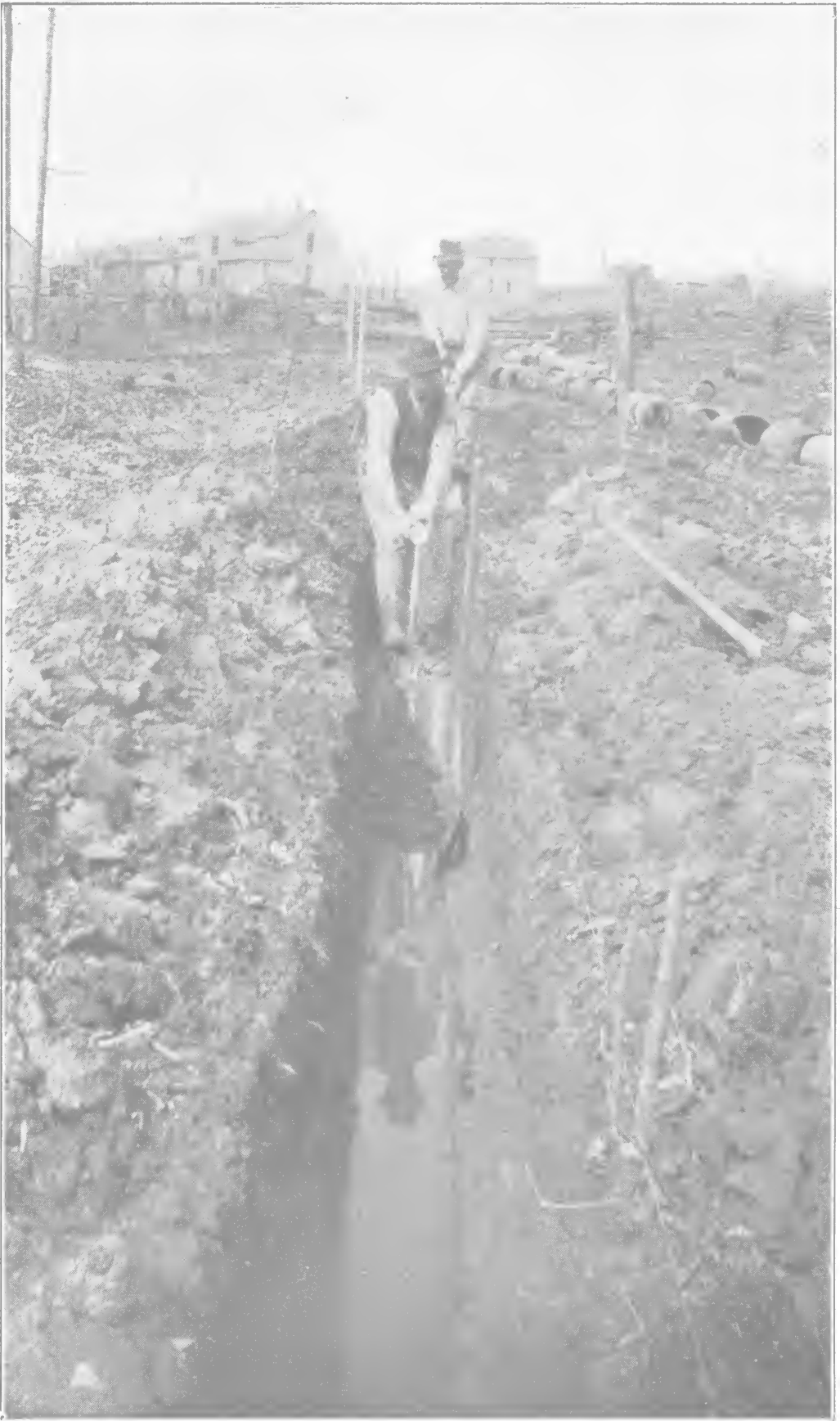
DIGGING A DITCH FOR TWELVE-INCH DRAIN-TILE.
