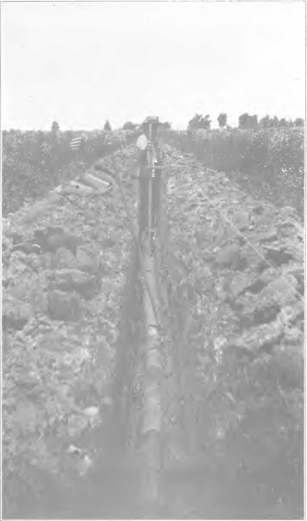
A FOUR-INCH LATERAL DRAIN.
