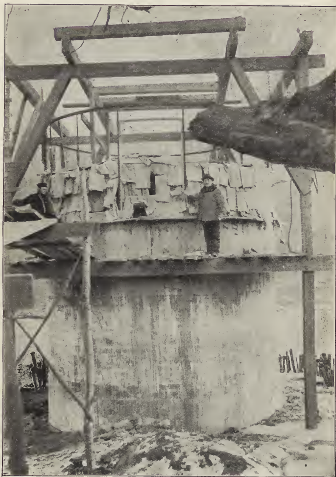
Fig. 154.—Construction of Intake Tank, LaSalle, Ill.
