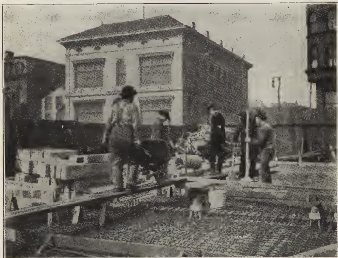
Fig. 81.—Concreting Floors in Winton Garage, Chicago.
