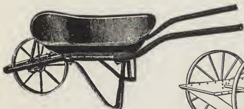
Fig. 88.—Iron Wheelbarrow for Handling Concrete.
