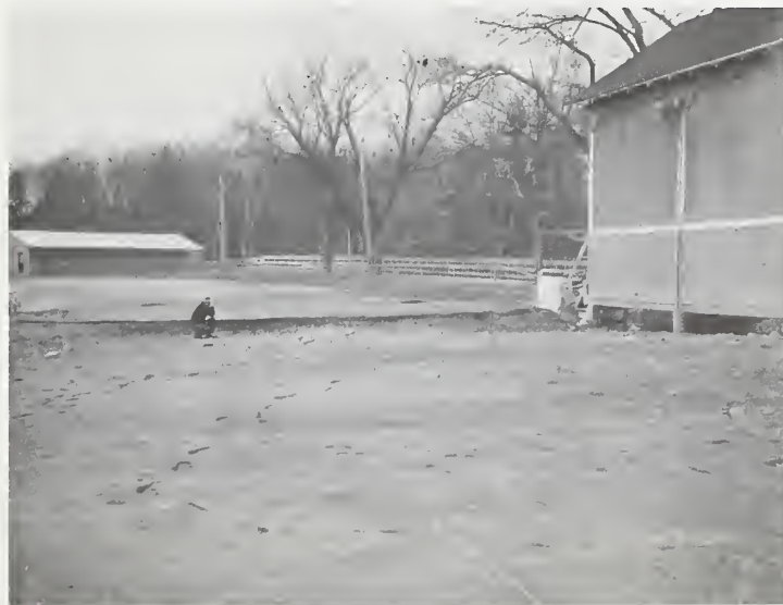
Union Fairgrounds - This area suffers quite frequent flood damage. The top photo, taken in front of the grandstand, shows the estimated elevation of the 100-year flood to be 45.4 feet NGVD or 5.3 feet above the track. The lower photo shows damage to the track caused by the spring 1984 flood, estimated to be approximately a 20-year event. (SCS photos)
