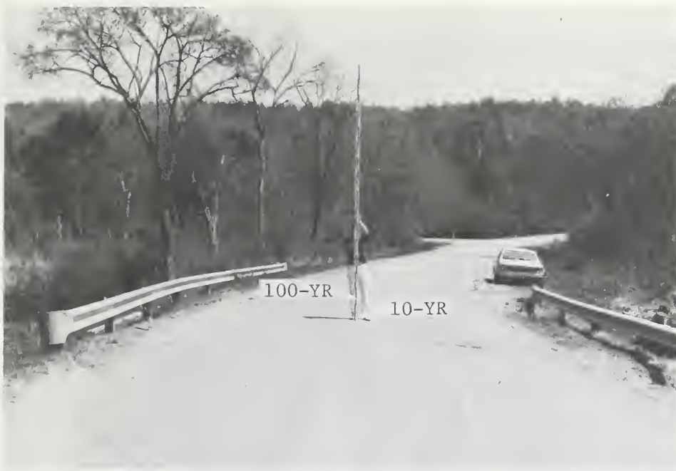
Medomak River, Shepard Hill Road, cross section M14B - The 100-year flood is estimated to be at elevation 149.4 feet NGVD or 1.3 feet over the road. (SCS photo)
