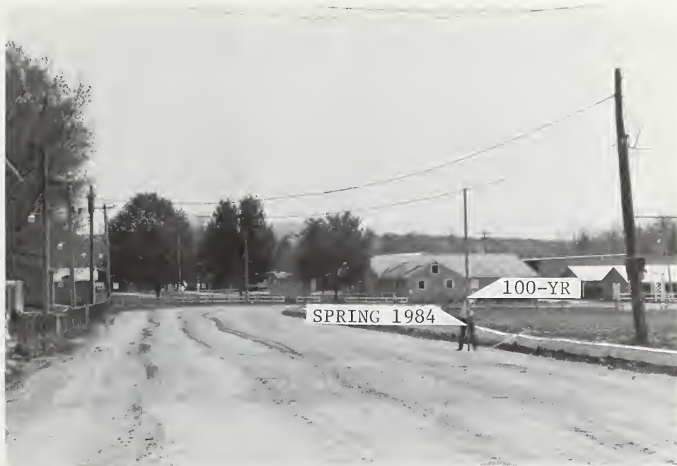
Union Fairgrounds - This area suffers quite frequent flood damage. The top photo, taken in front of the grandstand, shows the estimated elevation of the 100-year flood to be 45.4 feet NGVD or 5.3 feet above the track. The lower photo shows damage to the track caused by the spring 1984 flood, estimated to be approximately a 20-year event. (SCS photos)
